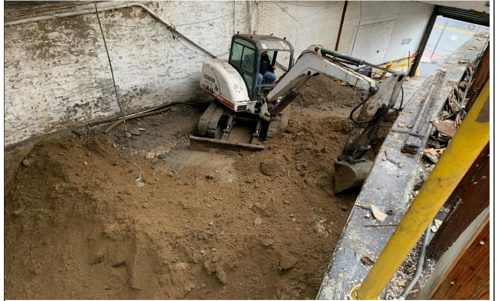
Photo 1 – View of backfilling of UST excavation from the non-impacted soil pile
