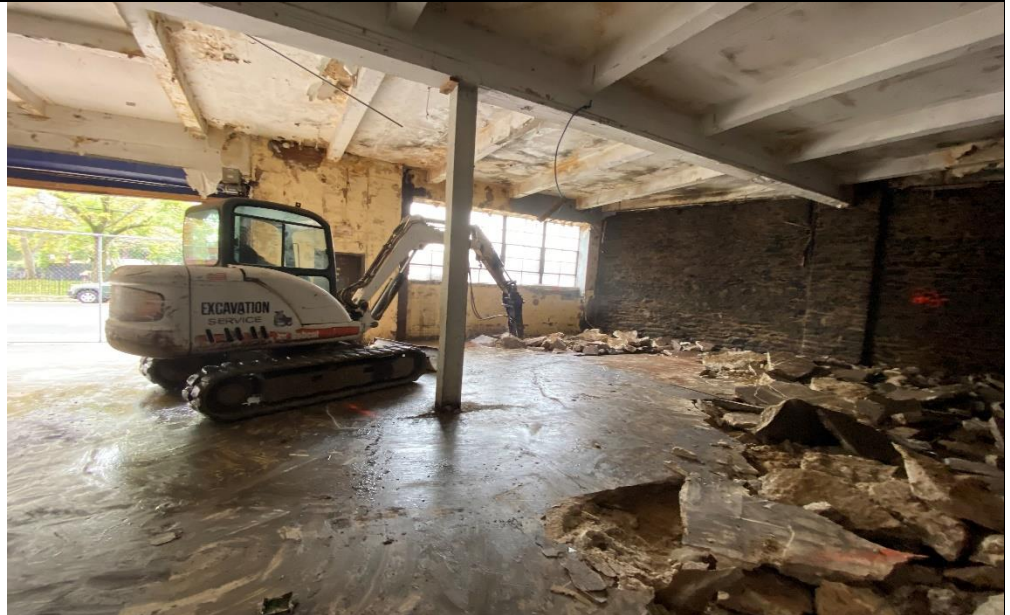
Photo 1 – View of slab demo on ground floor
