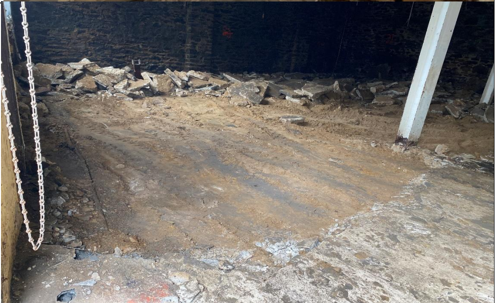
Photo 2 – View of broken up slab cleared, exposed soil
