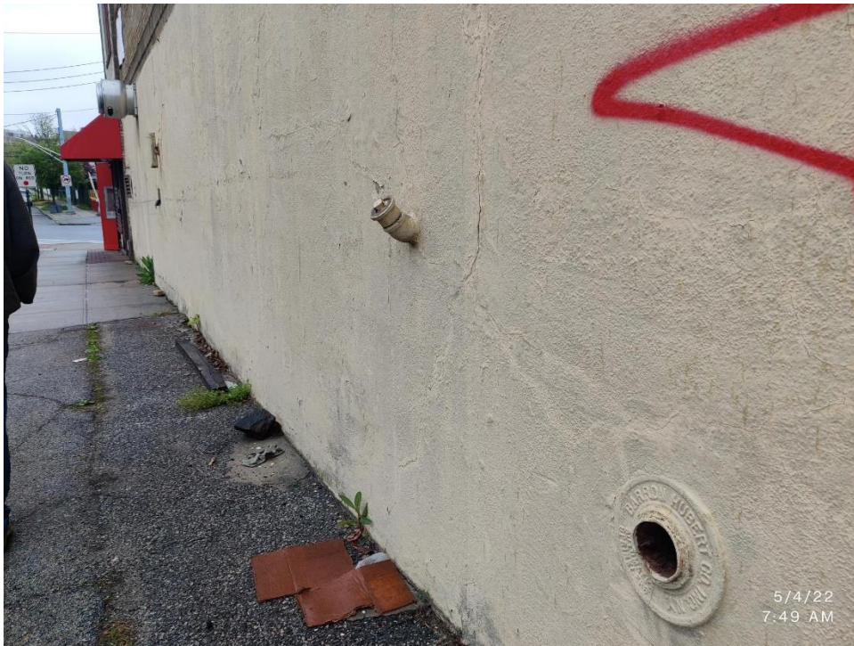
Photograph No. 7: View of fill port on east side of building
