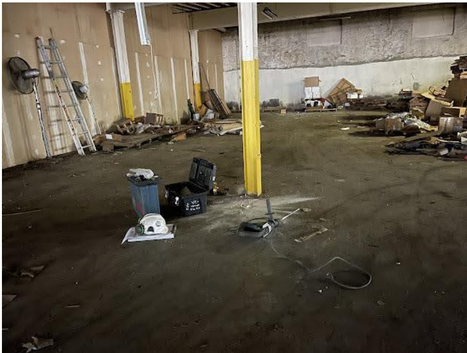
Photograph No. 5: View of typical installation of soil vapor monitoring pin setup
