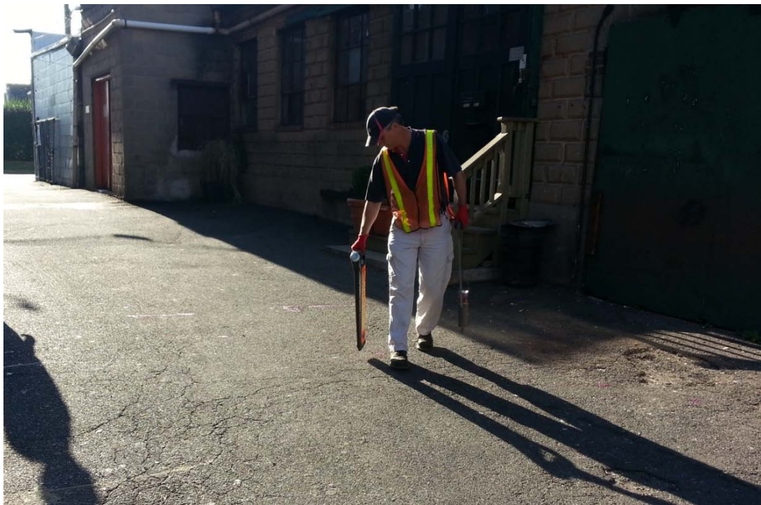
Geophysical survey technician clearing proposed boring locations for underground utilities.
