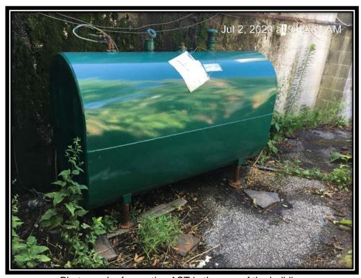
Photograph of an active AST in the rear of the building
