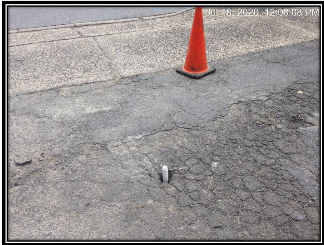
Photograph of the temporary 1-inch well installed in B-2 TW
