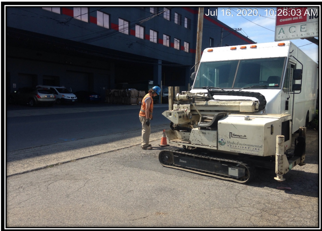
Photograph of the B-2 TW boring location
