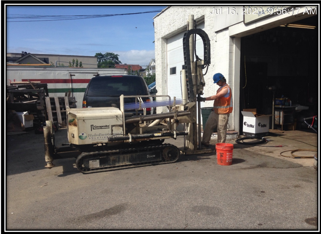
Photograph of boring B-1 being installed
