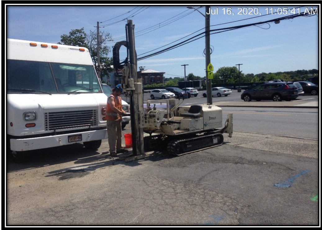
Photograph of the B-1 TW boring location
