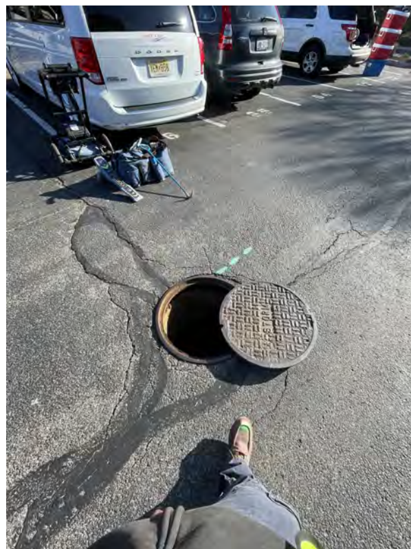
Fig. 4 : All storm structures were opened and investigated
