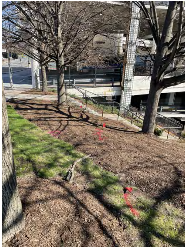
Fig. 1 : An image of the secondary electric running through the AOC
