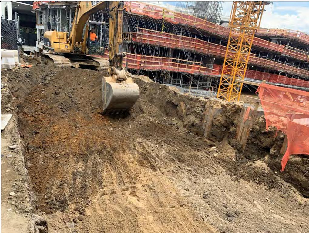
Photo 30: View excavation to clean endpoints outside the sheeting line A3 along Ferris Ave, 8/2/22
