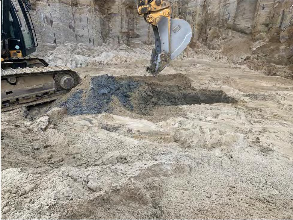
Photo 17: View of impacted soil found in grid F4, approximately 21 ft below original grade, 3/31/22
