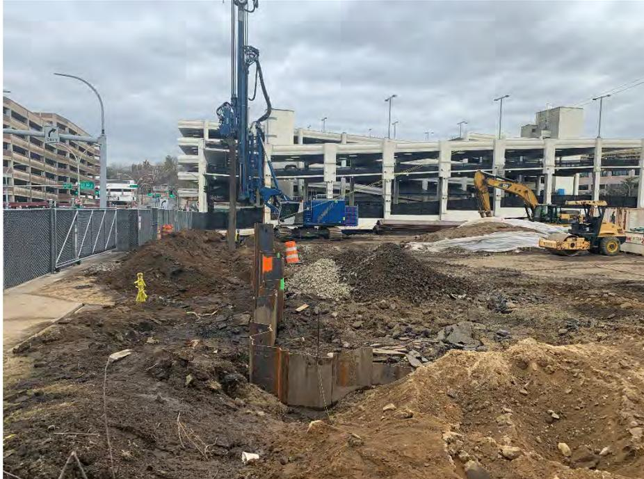
Photo 5: View of site face north, with sheet piles being installed along Ferris Ave, Grids A1-4, (2/17/22)
