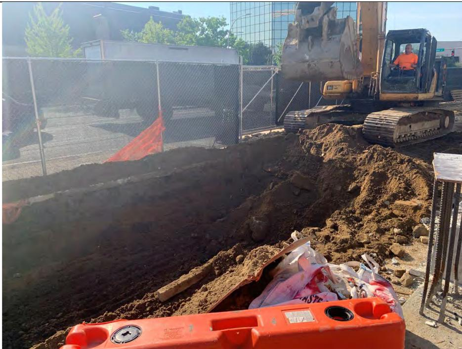
Photo 28: View of excavation to clean end points outside the sheeting line in F3, 7/21/22
