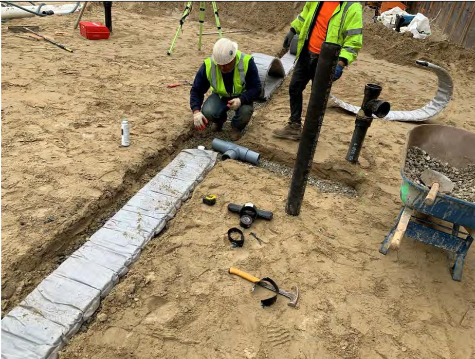
Photo 22: View of SSDS being installed in F3, 4/26/22
