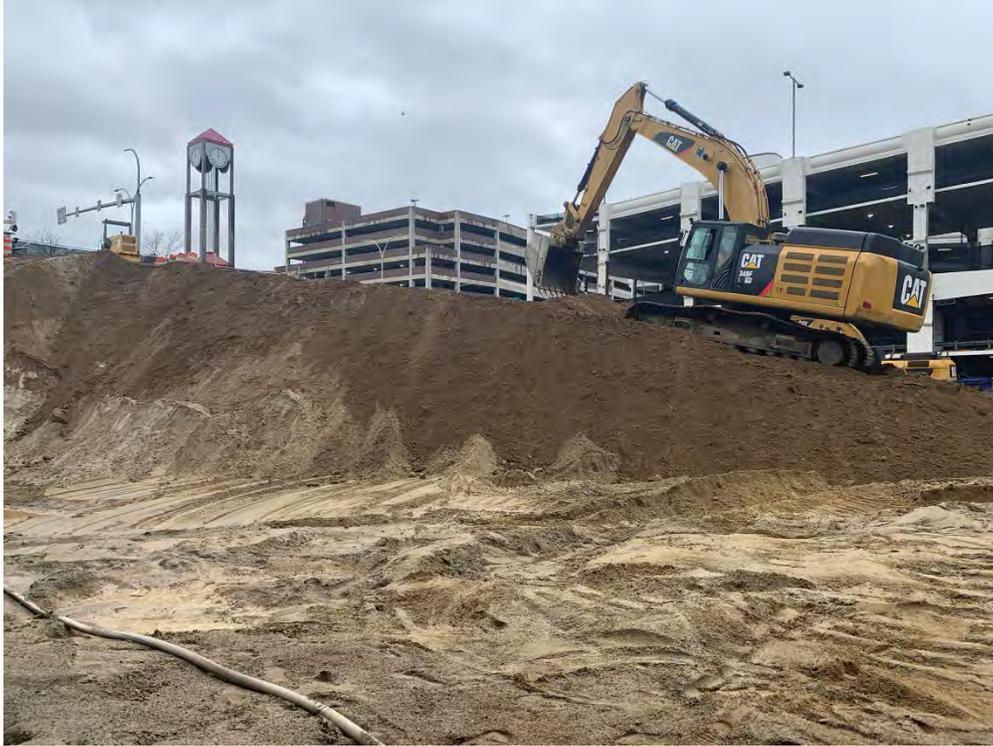
Photo 19: View of Soil Ramp constructed out of remaining A'4 material, 4/6/22
