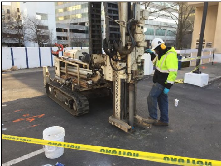
Photograph 3: Installation of 3.75-inch O.D. hollow casing at SB-14 for the installation of MW-7.
