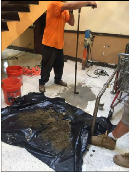
Photograph 1: Advancing SB-7 using hand auger.
