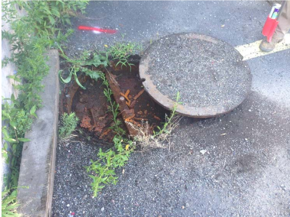
One of the manholes with the cover removed. Another cover was located beneath the soil.
