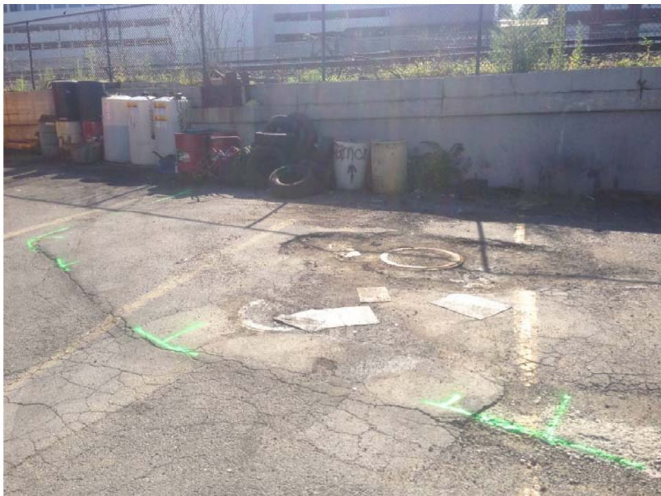
The geophysical survey marked out the large concrete anomaly which encompassed the manhole covers in the eastern portion of the site.
