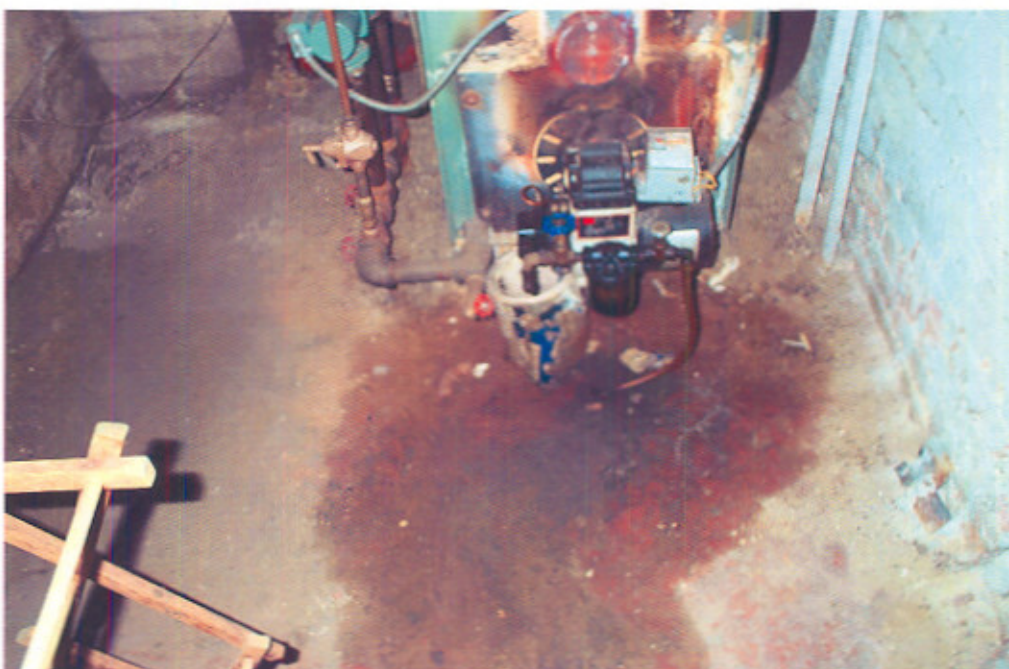
4. Minor surface staining near boiler at 330 South Street
