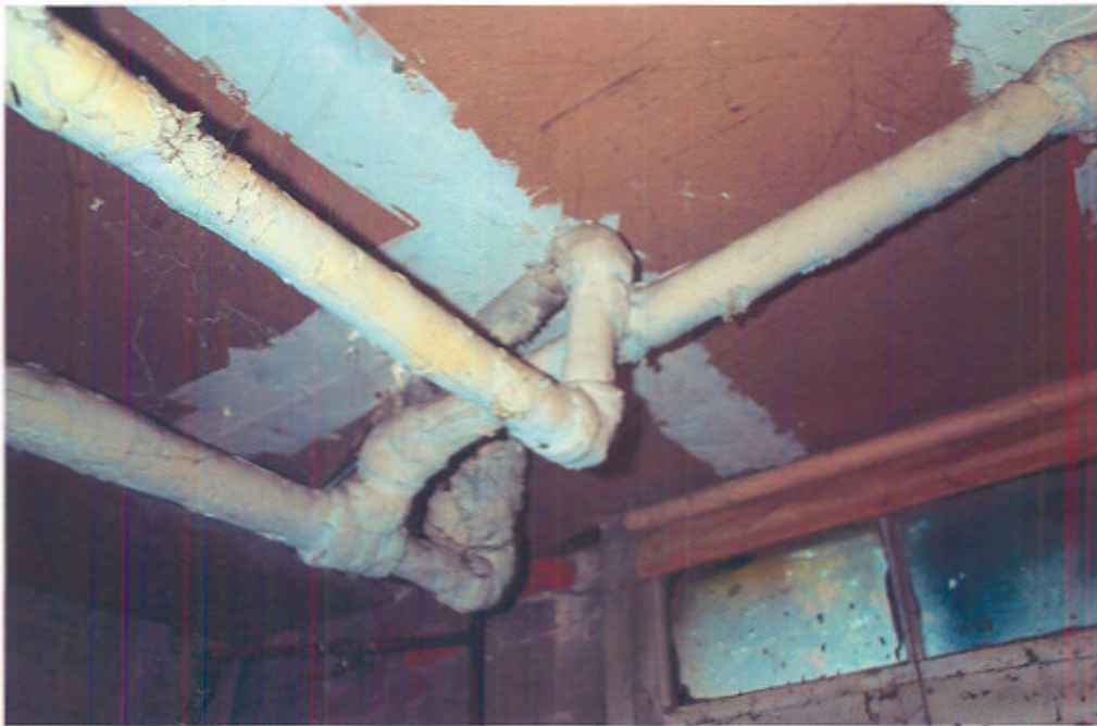
5. Suspect ACM pipe insulation at 330 South Street
