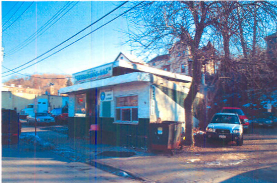
3. Subject property, looking northeast from Railroad Avenue
