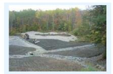
Designs for backfilling, grading and stabilizing a 3-acre basin affected by mining waste at the Elizabeth Mine NPL site in South Strafford, Vermont, included intent to mirror the site's natural contours and drainage patterns. The fully graded surfaces were seeded with native plant species that target Vermont state conservation and wildlife goals.
