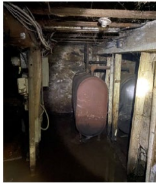
View of ASTs in the basement of 16 South Main Street
