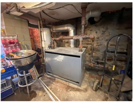
Photograph 9 – View of natural gas fired boiler and natural gas hot water heater in the cellar of 2 South Main Street.
