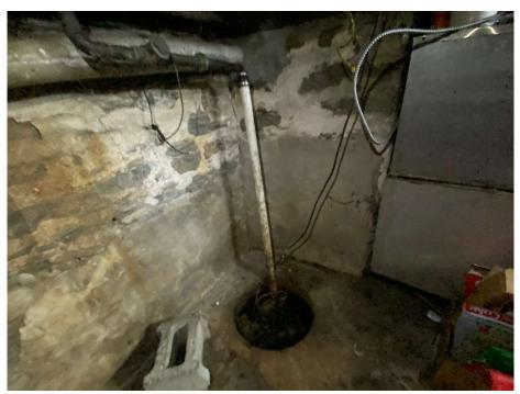
Photograph 12 – View of sump pump within the southeastern corner of the cellar at 8 South Main Street.
