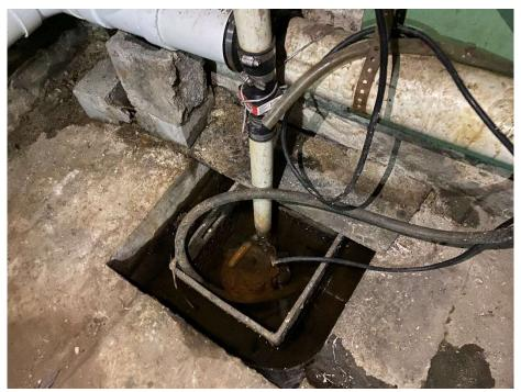
Photograph 18 – View of sump pump within the southeastern corner of the cellar at 106 Westchester Avenue.
