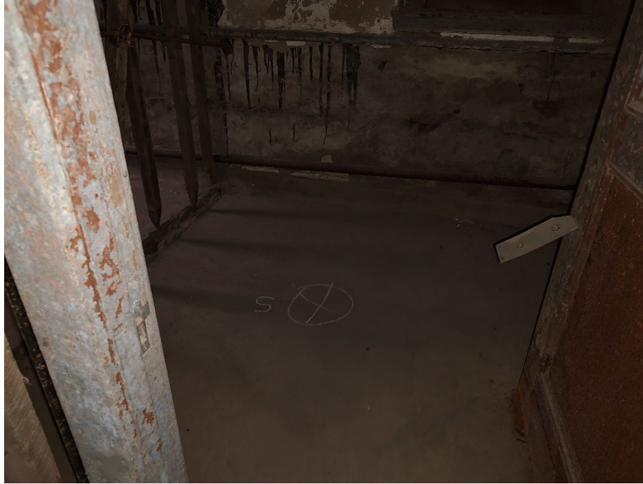
Photo 6 – View of a proposed boring location within the lowest accessible level of the theater along the north rear wall.
