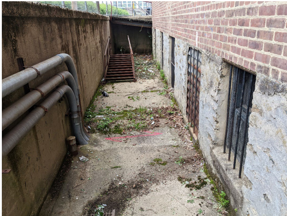
Photo 5 – Multiple live electrical lines were detected at the rear of the theater building and within accessible areas in the theater, though the lowest level was inaccessible due to flooding.
