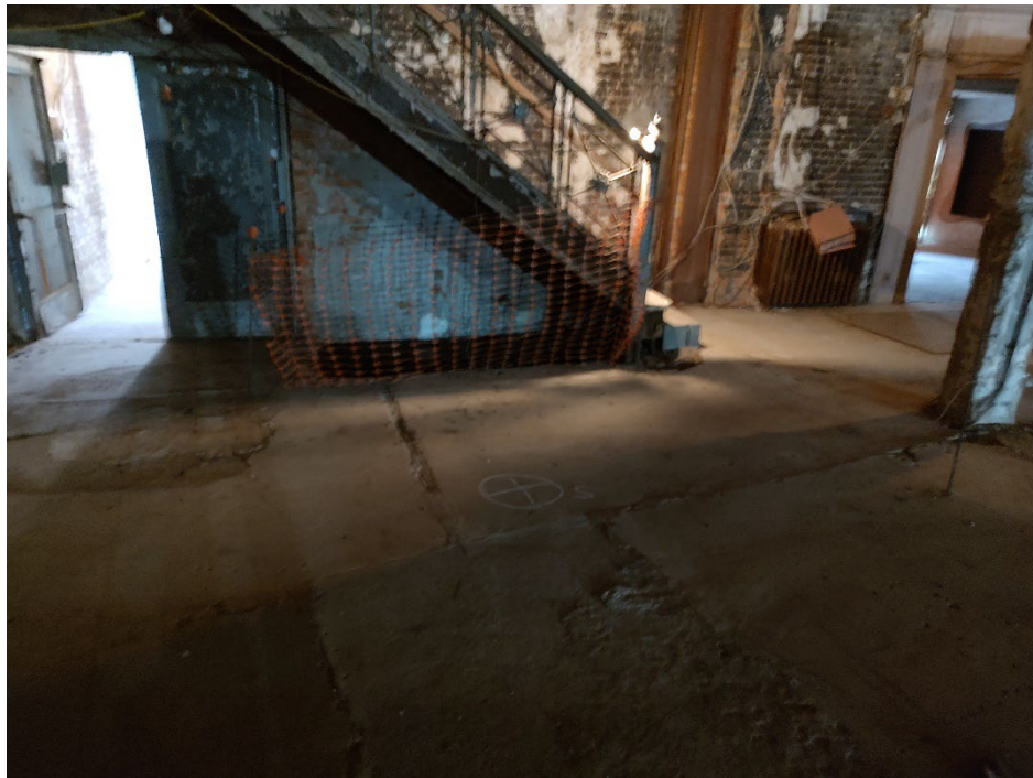
Photo 5 – View of a proposed boring location within the theater main level.
