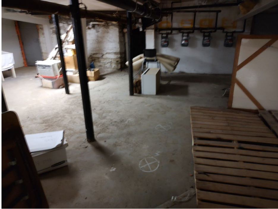
Photo 2 – View of the basement beneath #128 showing a proposed soil boring and temporary well.
