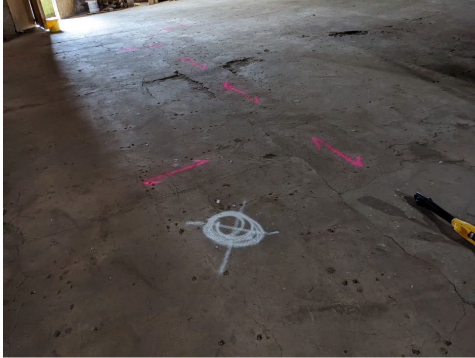
Photo 4 – View from within the Theater showing a proposed boring location in close proximity to multiple subgrade utilities.
