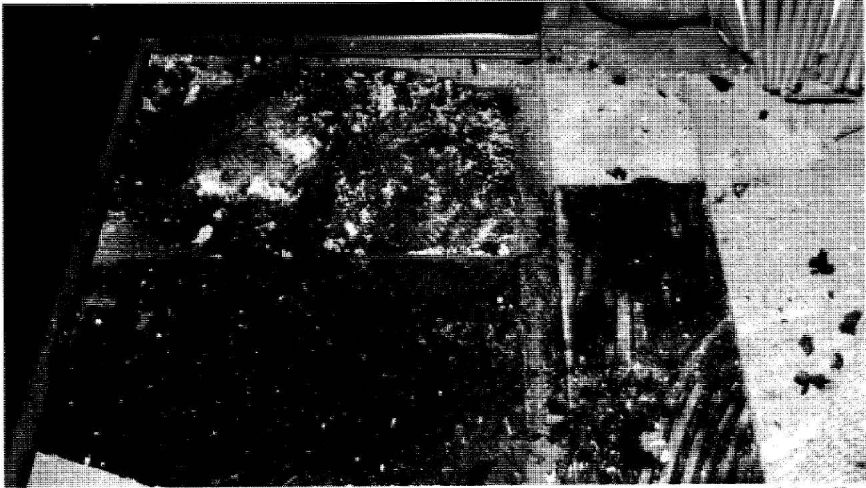
This picture shows the three layers of floor tiles found to be present on the first floor of the office building area.
