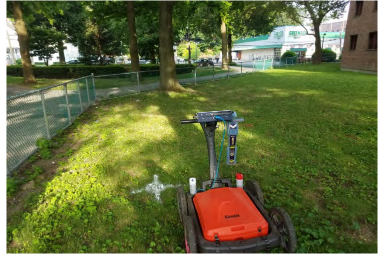
Photograph 2. Cleared boring location for SB-2.
