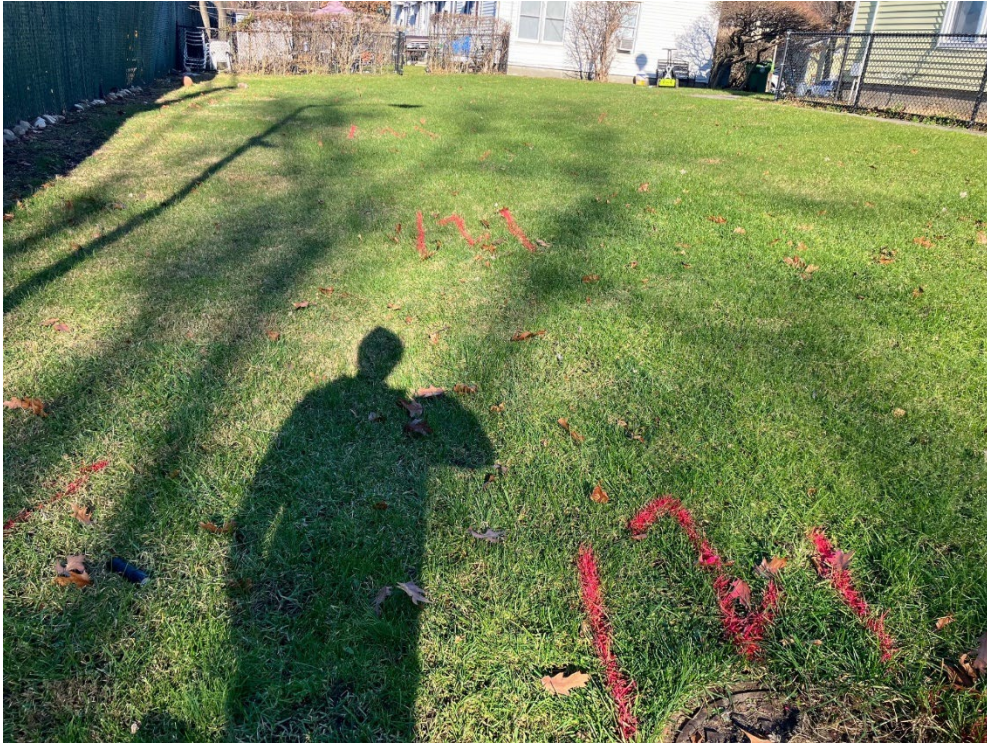
Photo 4 – View of the proposed soil boring location behind residence 10D. Within this area, a sanitary manhole and line was detected and avoided during drilling.
