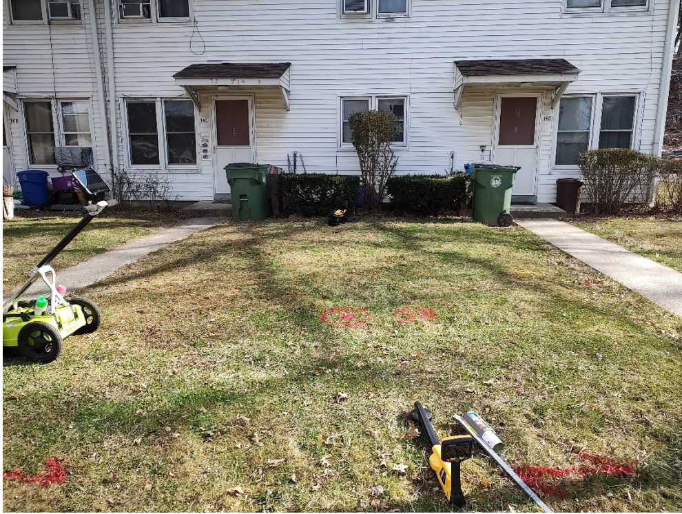
Photo 2 – View of the proposed soil boring locations within the area in front of residence 14D. Multiple subsurface anomalies were detected within this area including an electrical line and the soil boring location was adjusted accordingly.
