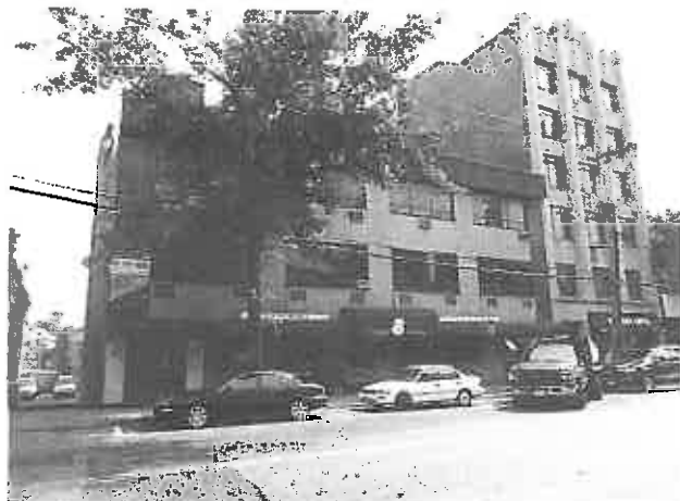
Southern side of the building facing southeast.
