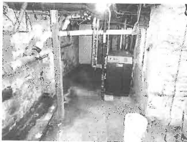
Interior view of the basement.
