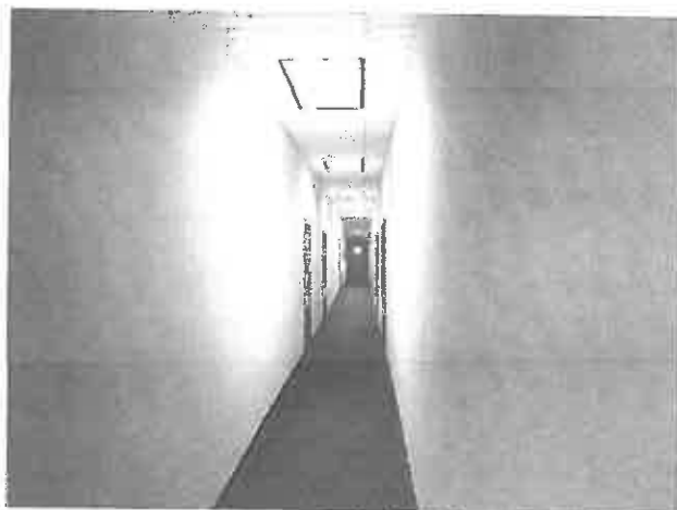
Typical view of the hallways in the office areas.
