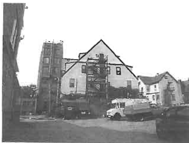
Northern side of the building facing south.
