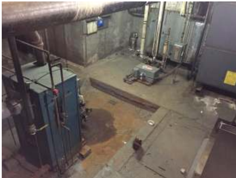
Photo 10: View of the basement – oil staining on the floors.
