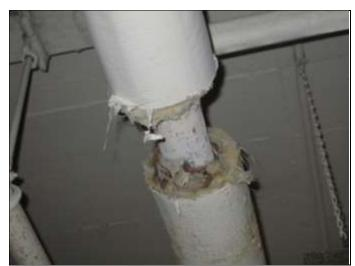
28. View pipe wrap, fiberglass visible.
