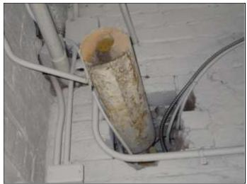
27. View of pipe wrap, fiberglass visible.
