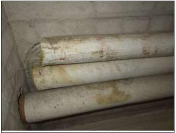
26. View of pipe wrap, fiberglass visible.
