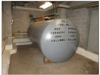
25. View of fuel oil AST located in basement.
