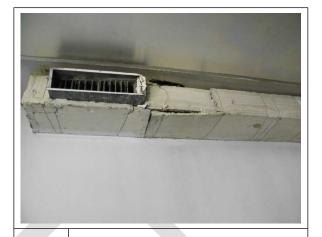
**10.** Insulation on ductwork (suspect ACM).
