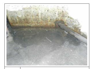
Oil staining on other side of wall from elevator equipment, basement.
