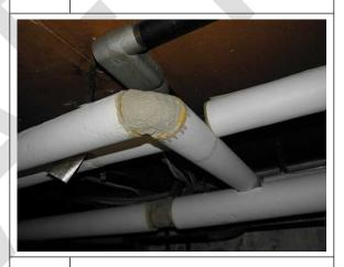
Mudded elbows on piping in basement (suspect ACM).
