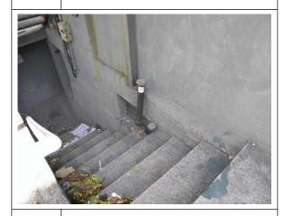
**6.** Fill pipe and vent on rear of building for fuel oil ASTs in building basement.
