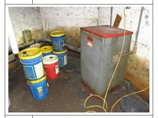
I2. Elevator equipment and buckets of hydraulic oil in basement. Note heavy oil staining on floor.
