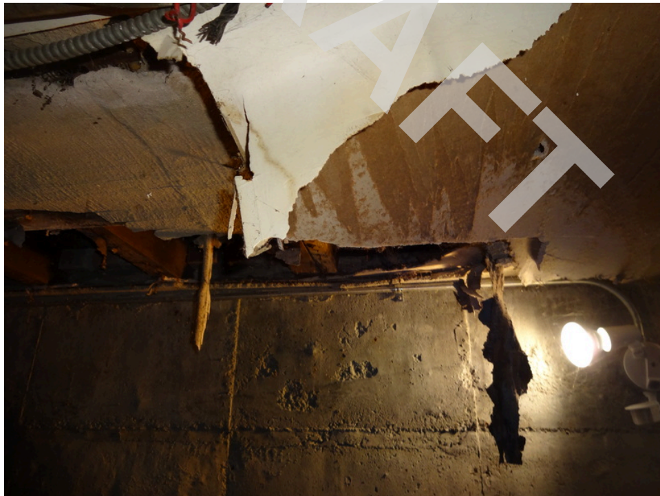
14. Damaged ceiling plaster in basement of pet store
