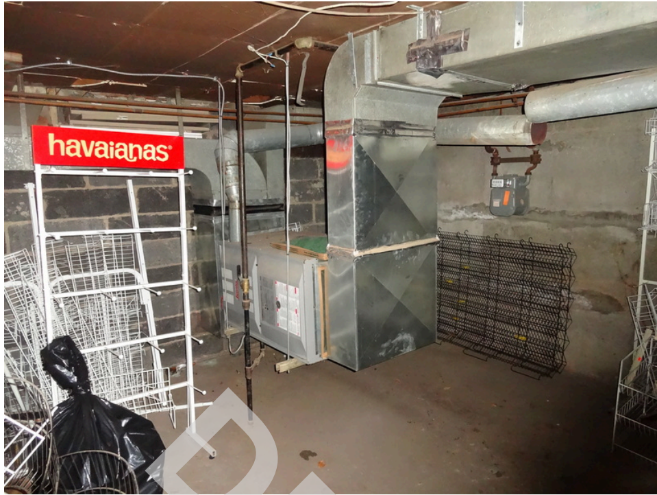
19. Natural gas furnace in basement of check cashing and currency exchange tenant space
