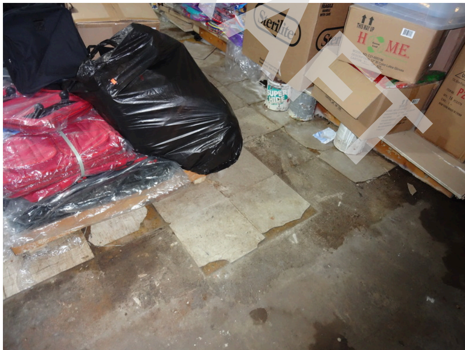
6. Damaged vinyl floor tile in basement of gift shop
