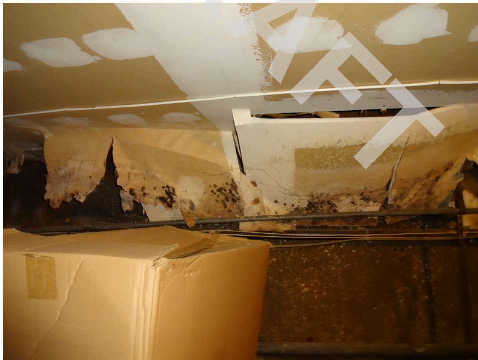
8. Damaged drywall and mold in basement of gift shop
