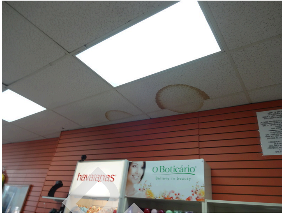
17. Stained ceiling tile at check cashing and currency exchange tenant space
