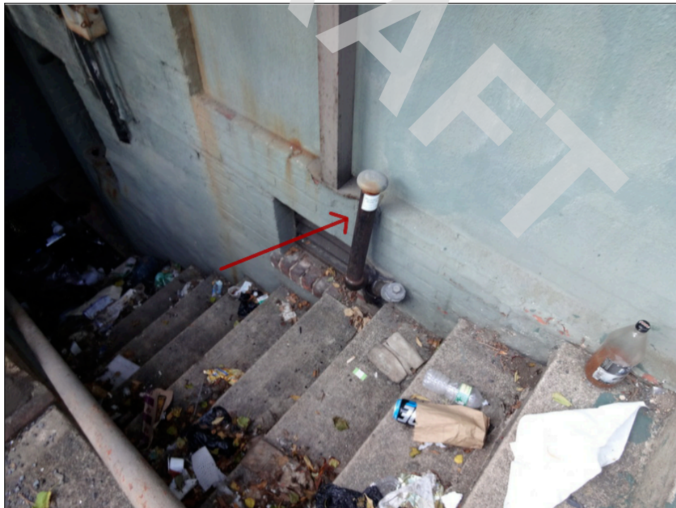
24. Fill port and vent pipe in rear of adjacent property to the southeast
