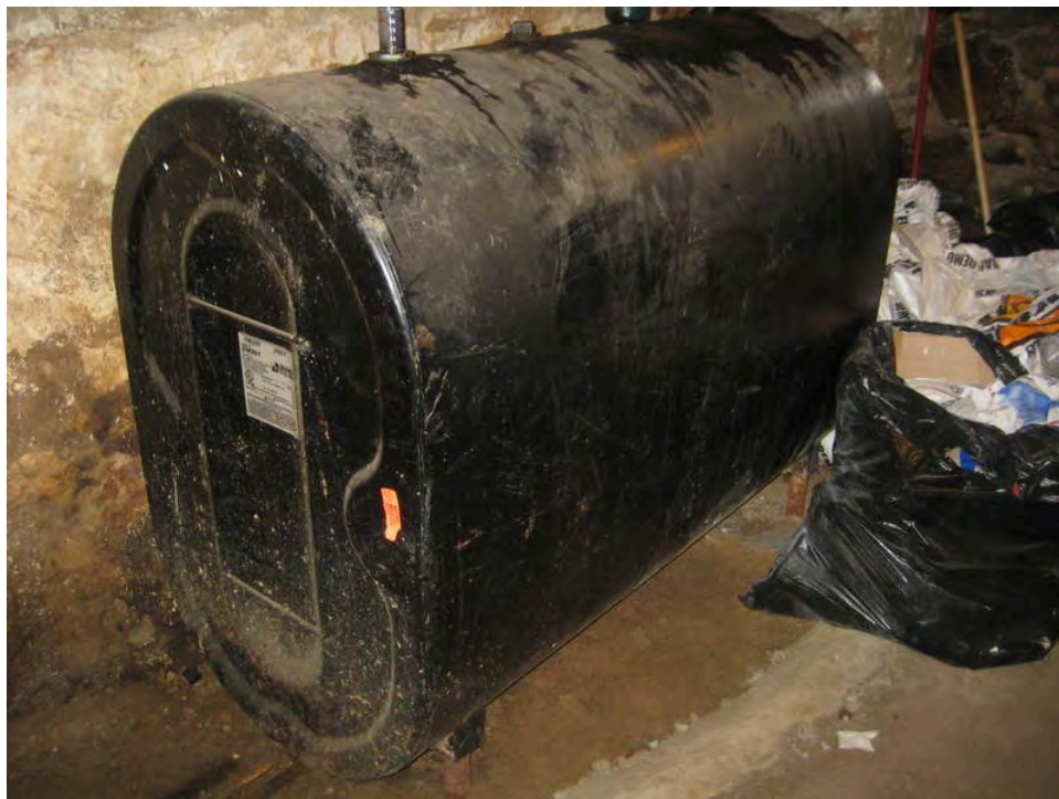
34. 275-gallon AST in basement of 485 Main Street.
