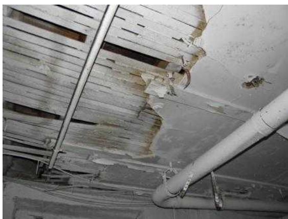
21. Lath and plaster system in basement ceiling.
