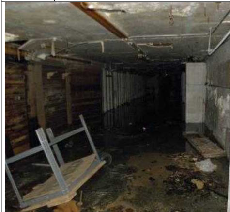
23. Flooded portion of basement of northern building.
