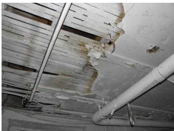
21. Lath and plaster system in basement ceiling.
