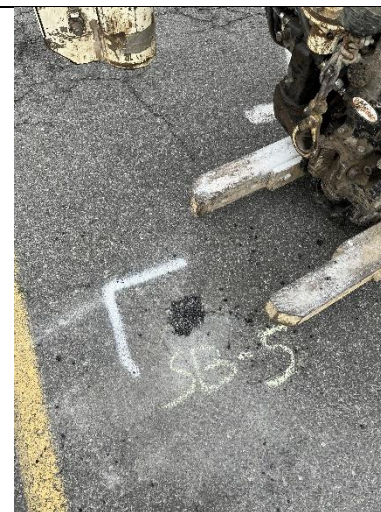
Photo 4 – View of completed boring. Borings were labeled with chalk, backfilled, and sealed with cold-patch asphalt.
