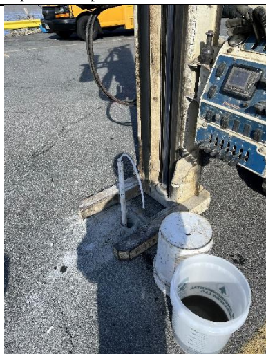
Photo 3 – Monitoring well TW-1, installed at soil boring location SB-7. Wells were 1" slotted PVC, which was purged of 3 well volumes and sampled.
