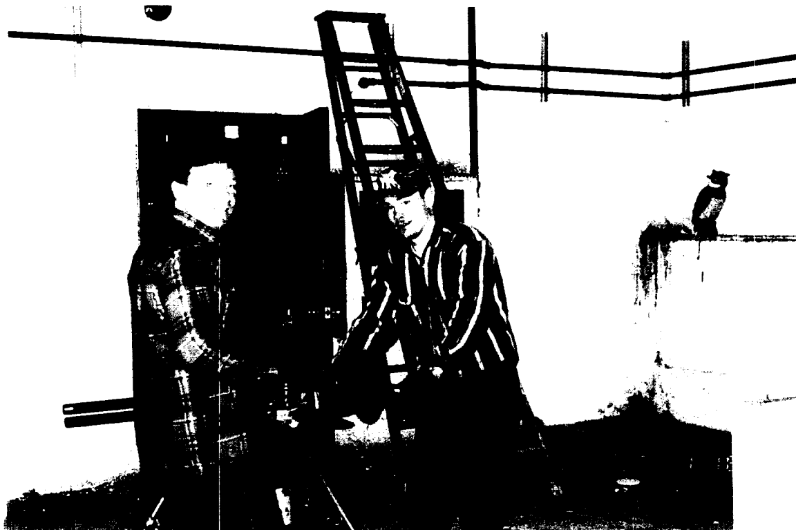
AST PIPING AND CONNECTION TO THE HEATING SYSTEM
