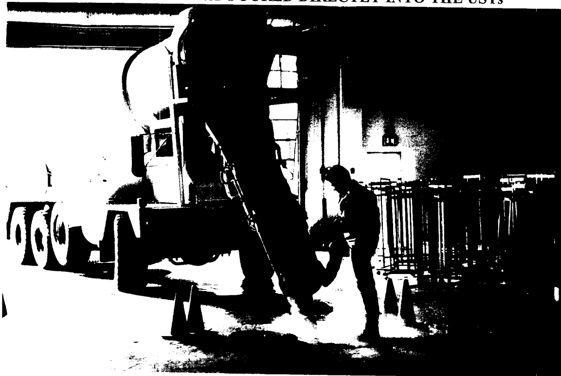
CONCRETE SLURRY POURED DIRECTLY INTO THE USTs
