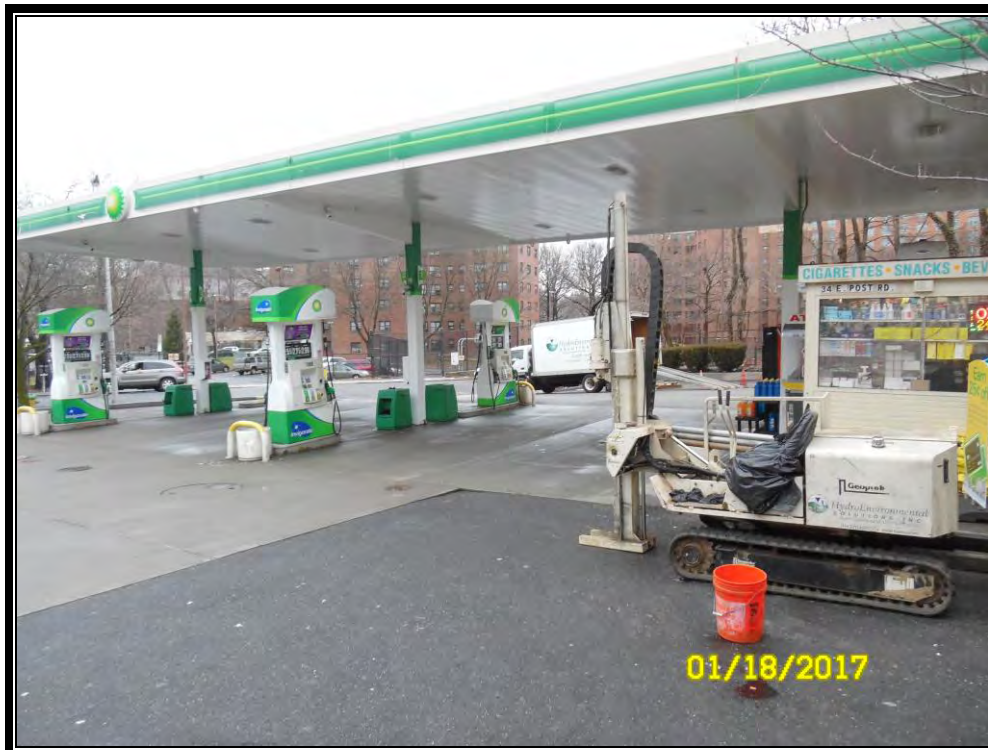
Photograph taken during drilling activities (GB-7)
