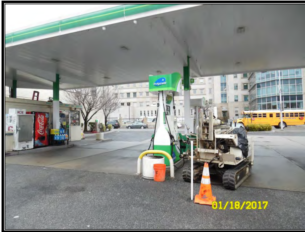
Photograph taken during drilling activities (GB-4)
