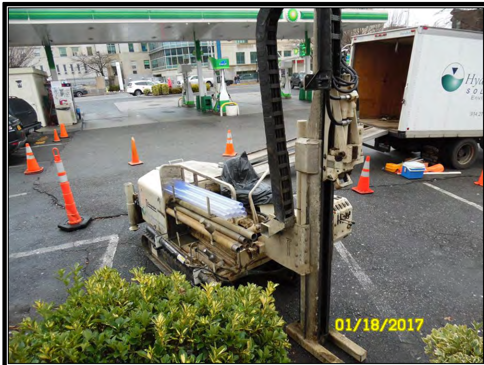
Photograph taken during drilling activities (GB-2)
