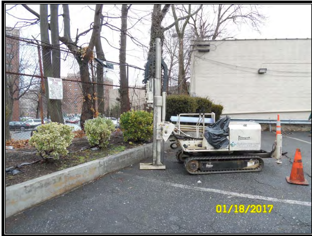
Photograph taken during drilling activities (GB-2)
