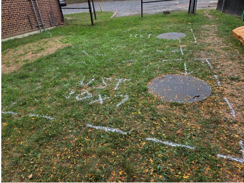
Photos 6 & 7 – View of two of the known USTs on site, marked in white to show the extent of the tanks and related piping.
