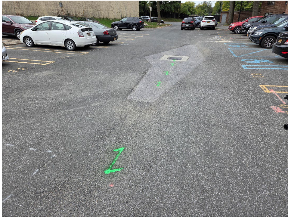
Photo 5 – Additional view of the drainage system.
