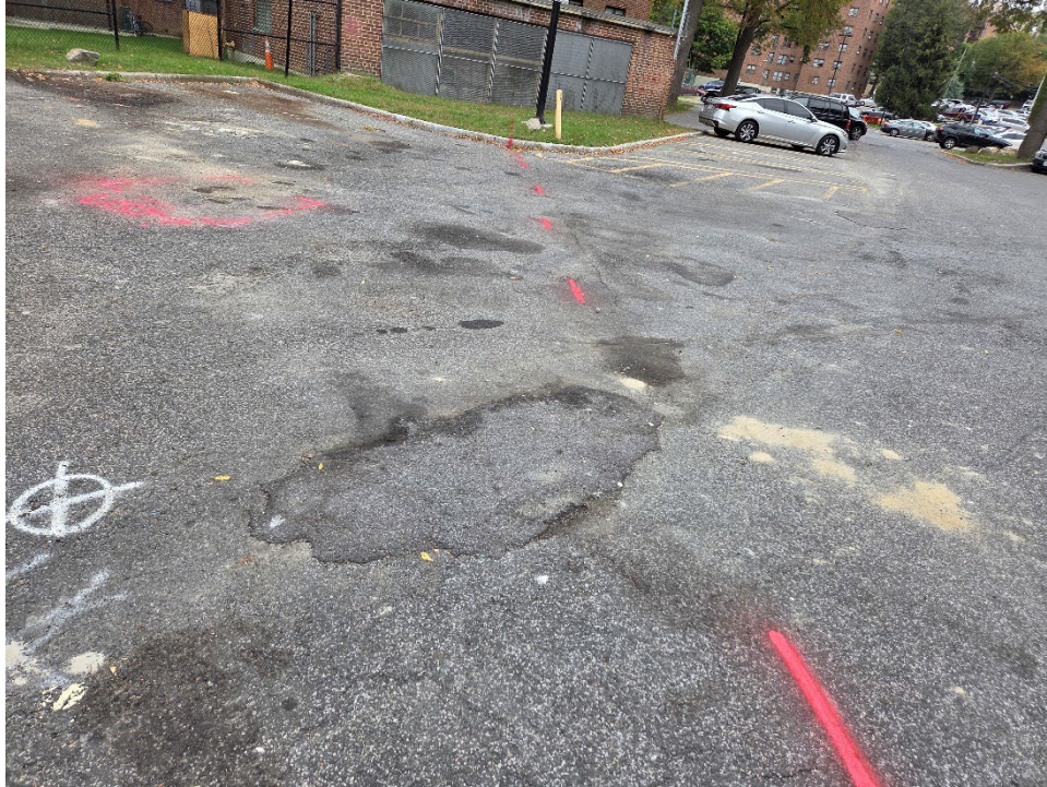
Photos 8 & 9 – Views of the areas investigated for suspected subsurface anomalies. The photo above shows the locations of two known USTs (white markings and arrow), while the subsurface detection below (marked in pink) was measured to be a square of approximately 3'x3' and not likely to be a UST. The additional area indicated by the arrow was investigated but no significant subsurface detections were found.
