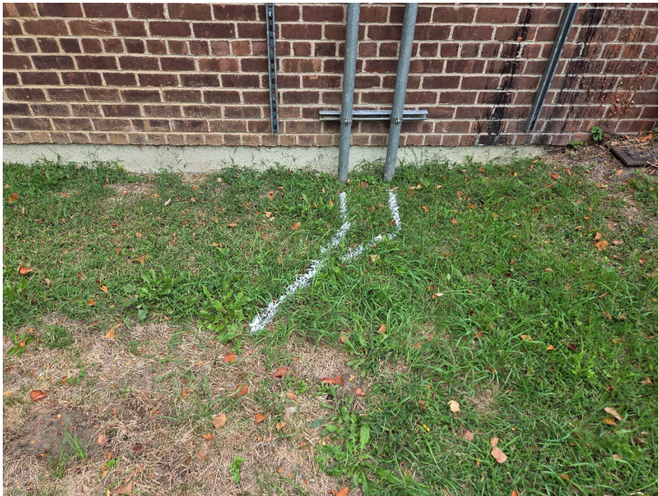
Photos 6 & 7 – View of two of the known USTs on site, marked in white to show the extent of the tanks and related piping.
