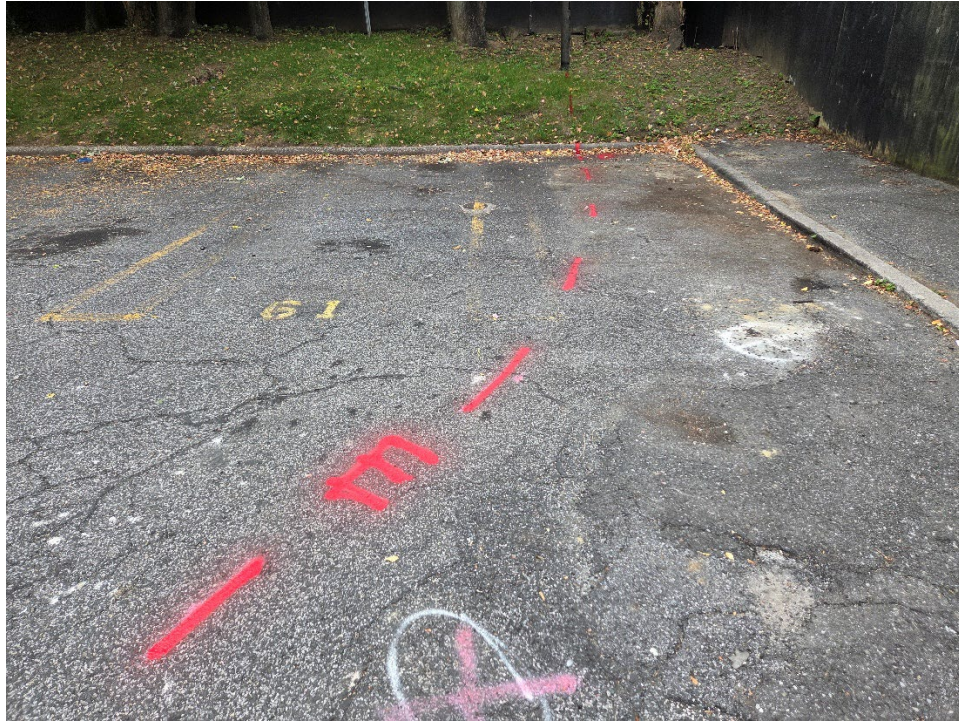
Photo 3- Additional electrical lines detected in the parking lot.
