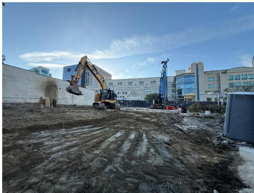
Piles installed along East Post Road
