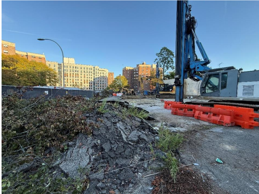
Concrete removal and site preparation
