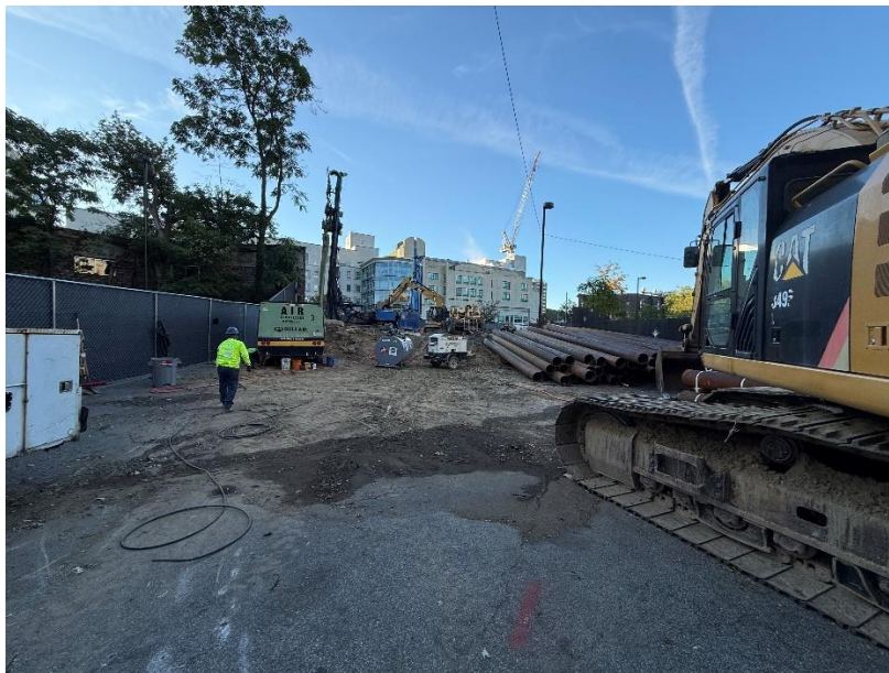
Pile and equipment delivery
