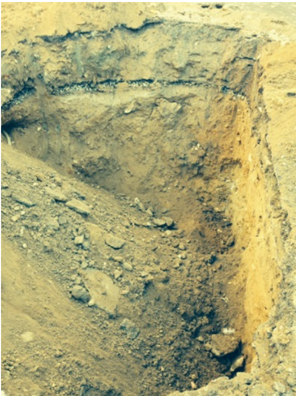
Photo 8- Excavation after UST removal (historical fill).
