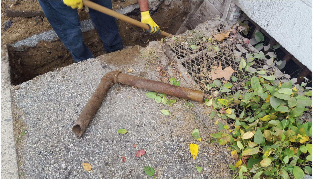
Photo 2 Removing the hanging fill and vent piping.
