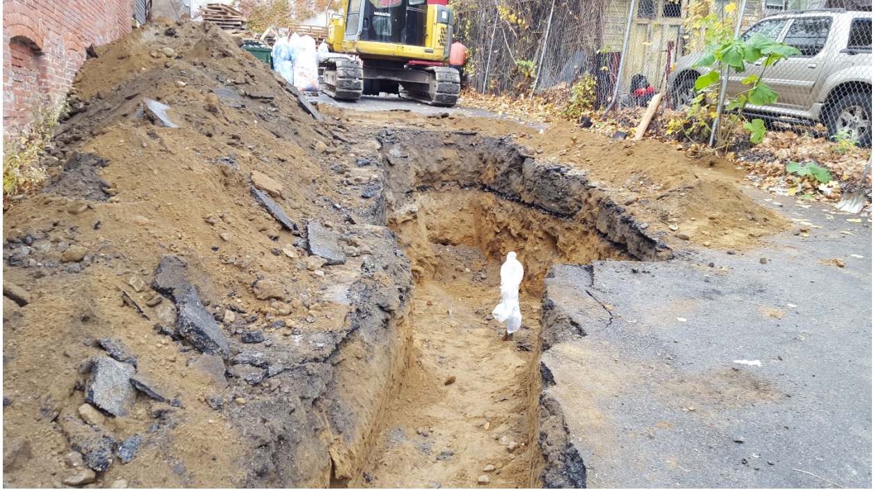
Photo 5-Exposing the top of the UST.
