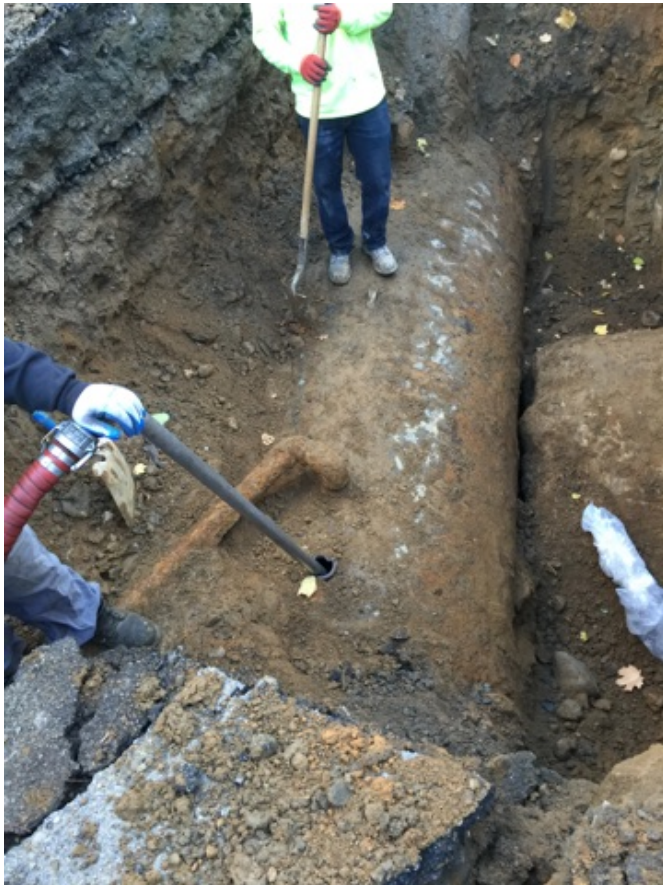
Photo 6 Pumping out the residual liquid for proper disposal.
