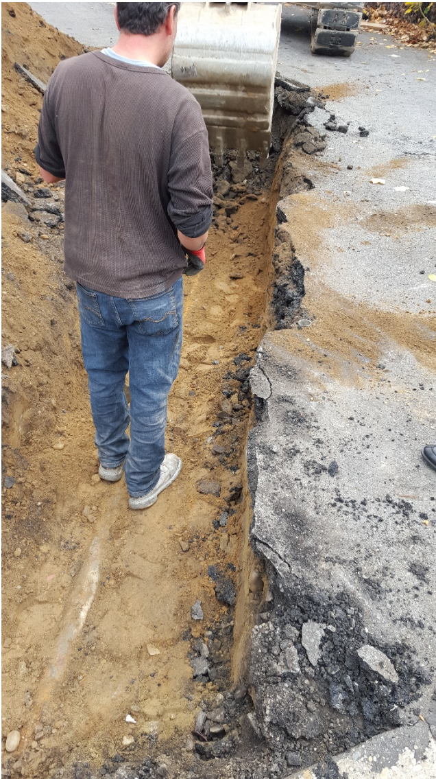
Photo 4 Tracing southern remote fill pipe easterly into building parking lot.
