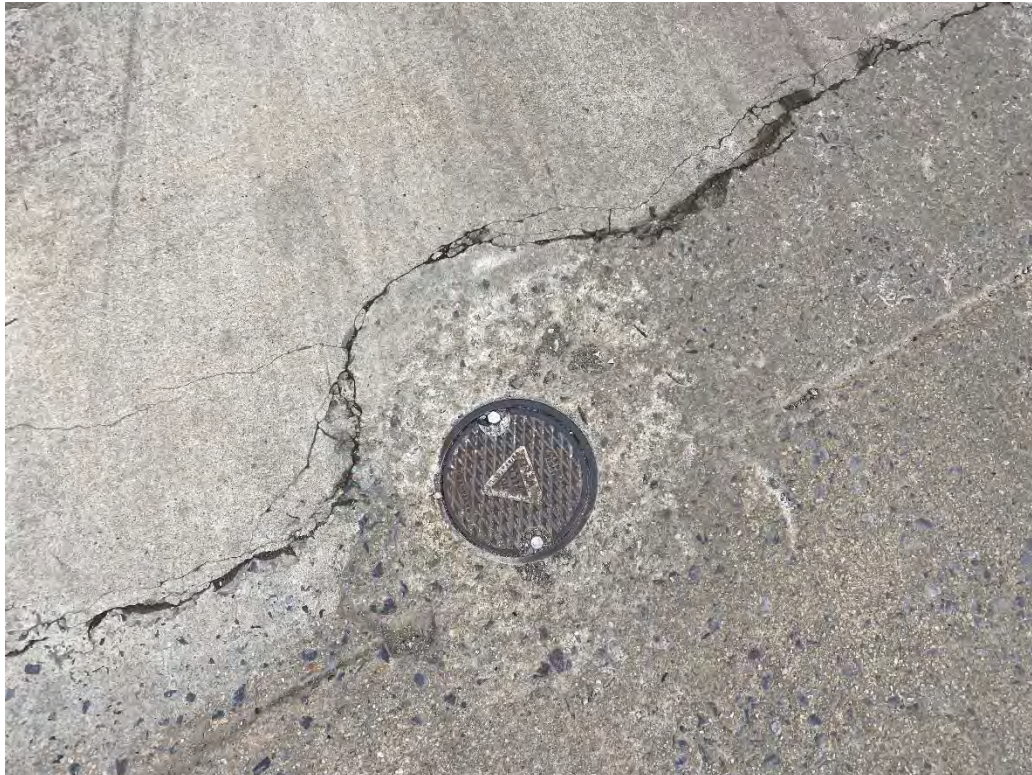
P.48 Monitoring Well Located in Southeastern Parking Lot
