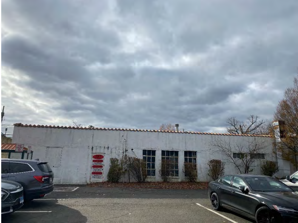
P.1 Northern façade of subject building
