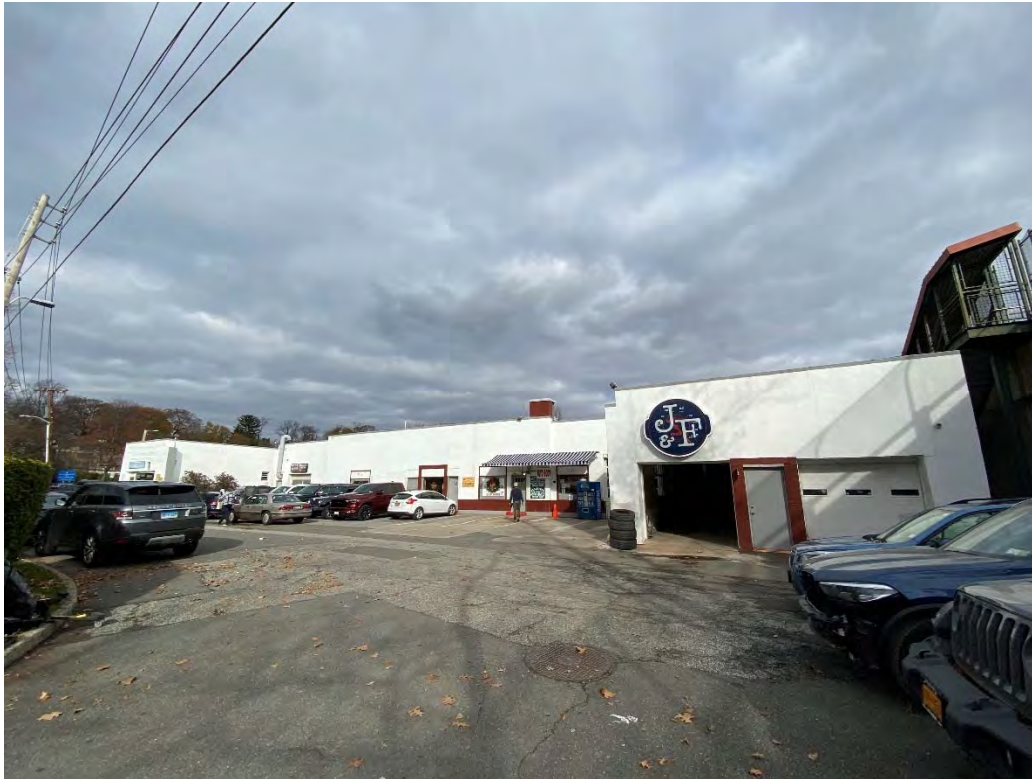
P.3 Southern façade of subject building
