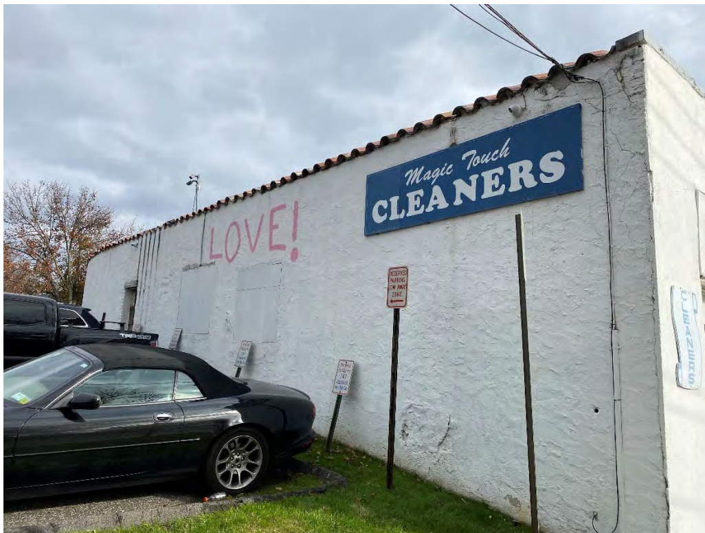
P.4 Western façade of subject building
