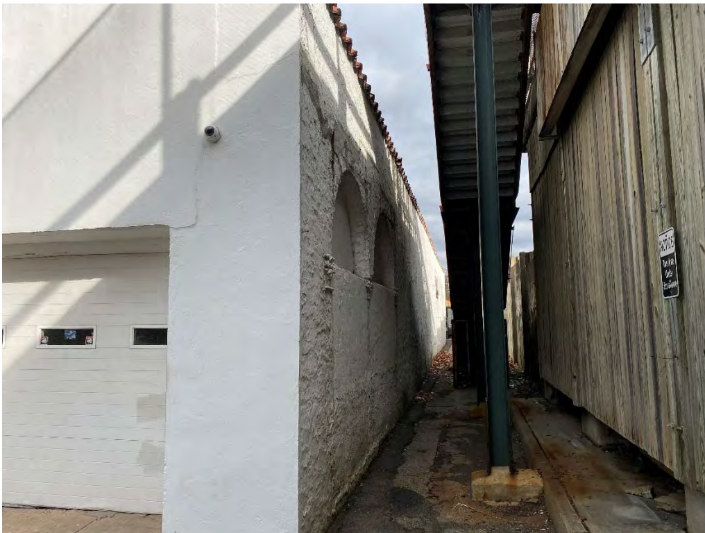
P.2 Eastern façade of subject building
