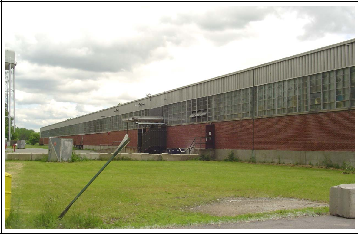
Photo #3 Description: Northern building façade.
