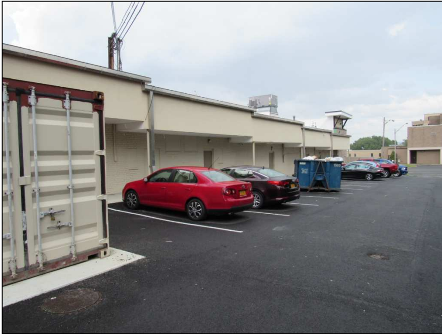
Southern wing of the building at 350 Northern Blvd., with the SVE Shed at far left.
