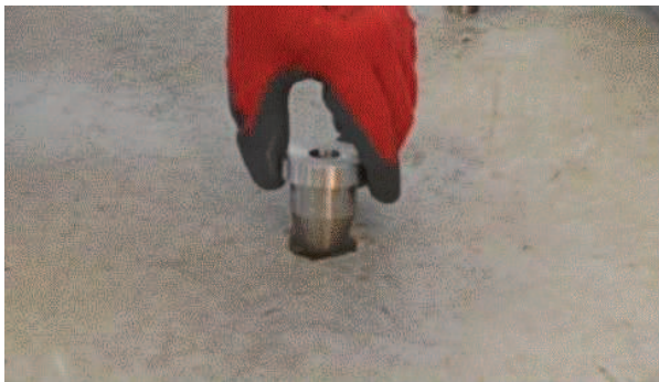
Figure 3. Installing the Drilling Guide.
