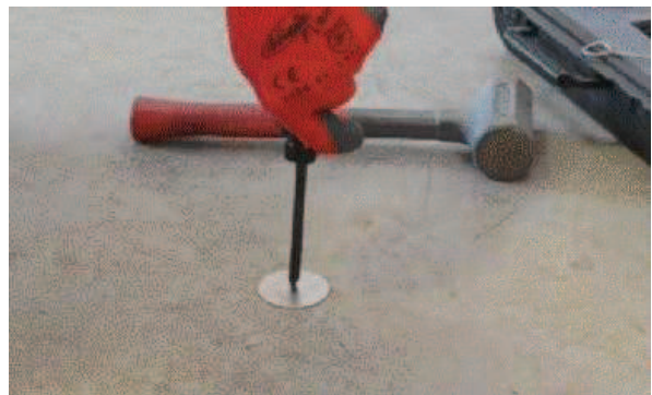
Figure 5. Tightening the Secured Cover.
