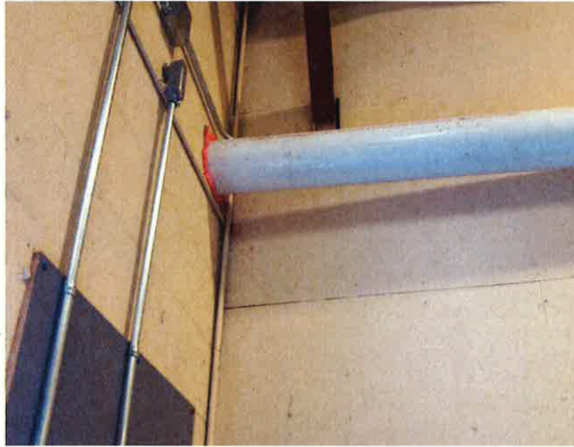
Photograph 17: View looking northeast at the 6-inch PVC final ducting system extending through the exterior wall in the left center of the photograph.
