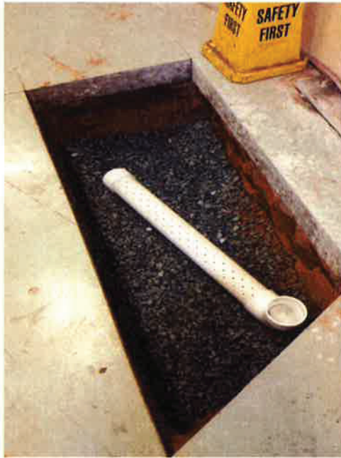
Photograph 5: View of 4-inch diameter PVC perforated duct installed into the soil vapor collection box at the EEA above an approximately 4-inch diameter layer of angular/sub-angular Type 2 stone below the duct.
