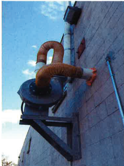
Photograph 18: View looking east at the Model PB-10A fan and emission system on the exterior of the Troy Belting facility. The duct is observed extending through the exterior wall in the right center of the photograph and is connected to the fan inlet.
