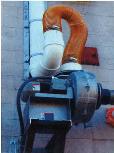
Photograph 19: Close-up view looking at the fan and emission system on the exterior of the Troy Belting facility. Flexible 6-inch duct connects to the 6-inch PVC “U” which will have a drain installed to remove the majority of condensation. The fan’s condensation drain is visible at the lower right.
