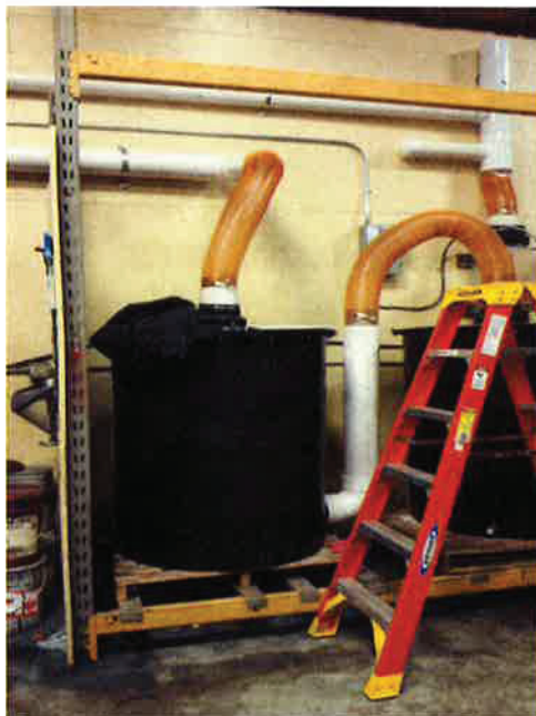
Photograph 16: View of the 6-inch PVC and flex ducting of the carbon treatment system. The 6-inch flex duct and PVC duct connecting the two G-10P canisters is observed in the right center of the photograph. The 6-inch flex duct and PVC duct from the outlet of the second G-10P carbon canister is in the left of the photograph.
