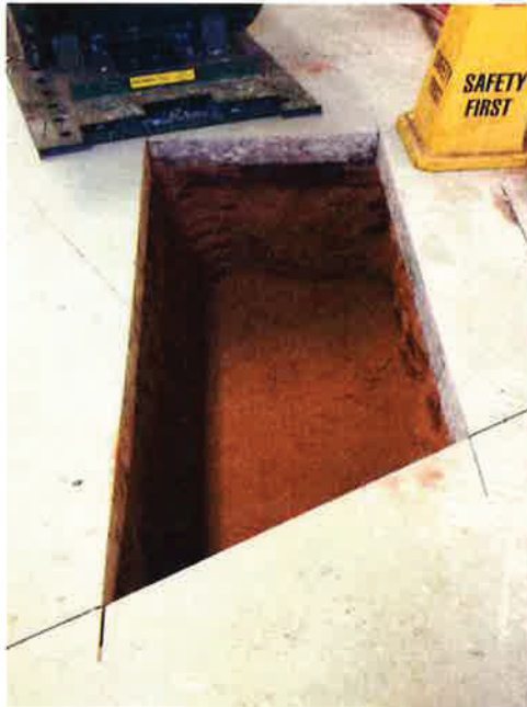
Photograph 3: View of the materials found in the WEA and EEA. Each withdrawal point had approximately 2 feet of materials excavated.
