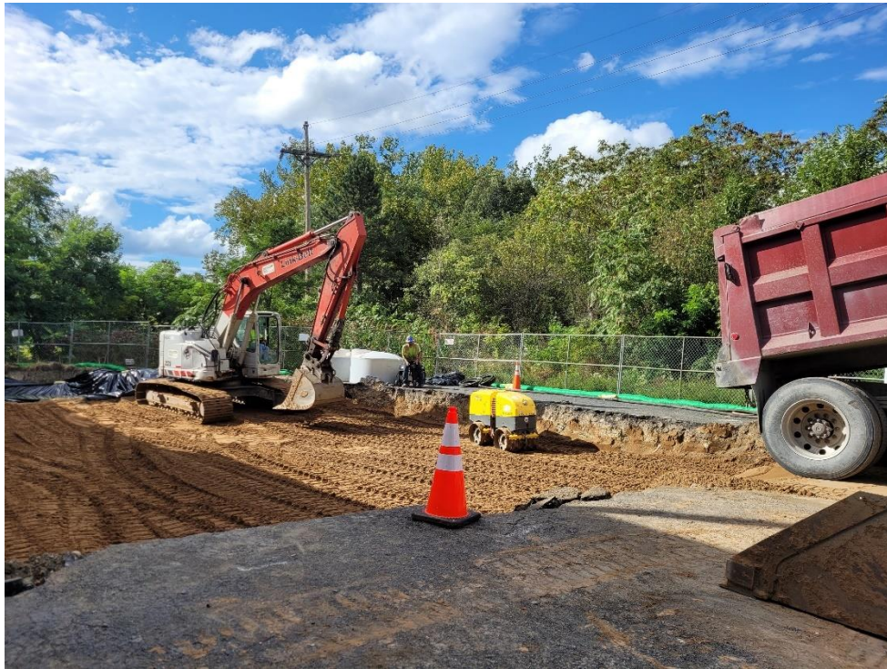
Photograph 31: Placement and compaction of approved backfill. View facing northwest. (Photo taken 9/24/21).
