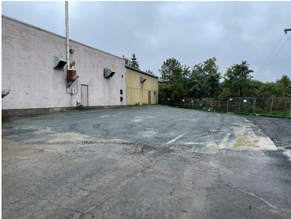
Photograph 33: Completed backfill of IRM excavation area with six inches of approved stone backfill. View facing west-southwest. (Photo taken 10/5/21).
