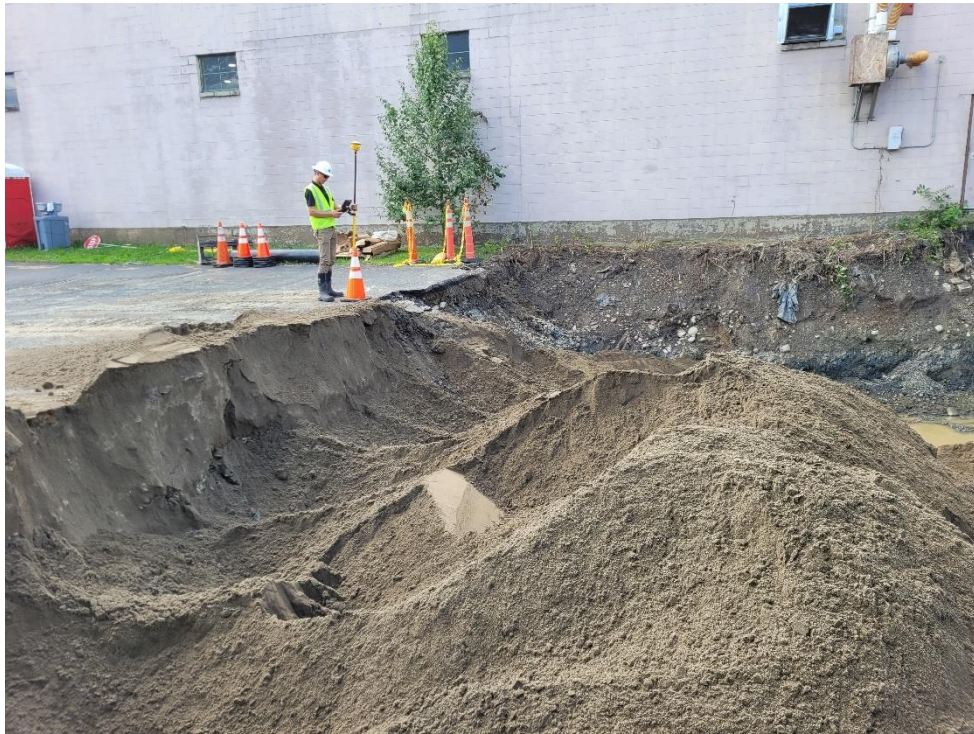
Photograph 27: GPS documentation of completed excavation limits. View facing south. ( Photo taken 9/21/21).
