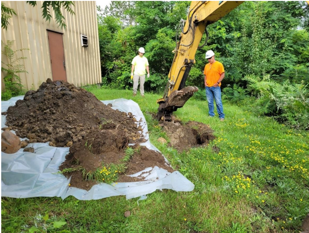
Photograph 1: Test Pit for collection of non-hazardous waste characterization sample. View looking west-southwest. (Photo taken 7/14/21).
