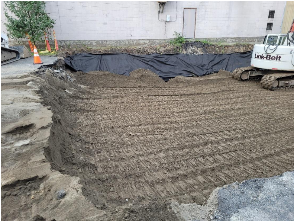
Photograph 30: Placement and compaction of approved backfill. View facing south. (Photo taken 9/22/21).
