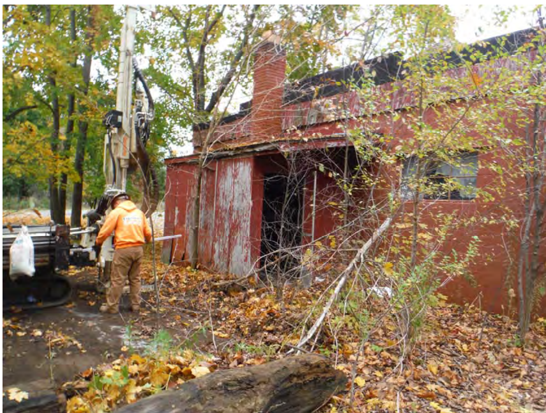
Photograph #3 – Advancement of soil boring SB-3 (monitoring well MW-3) at subject Property on October 20, 2015. Facing westerly.
