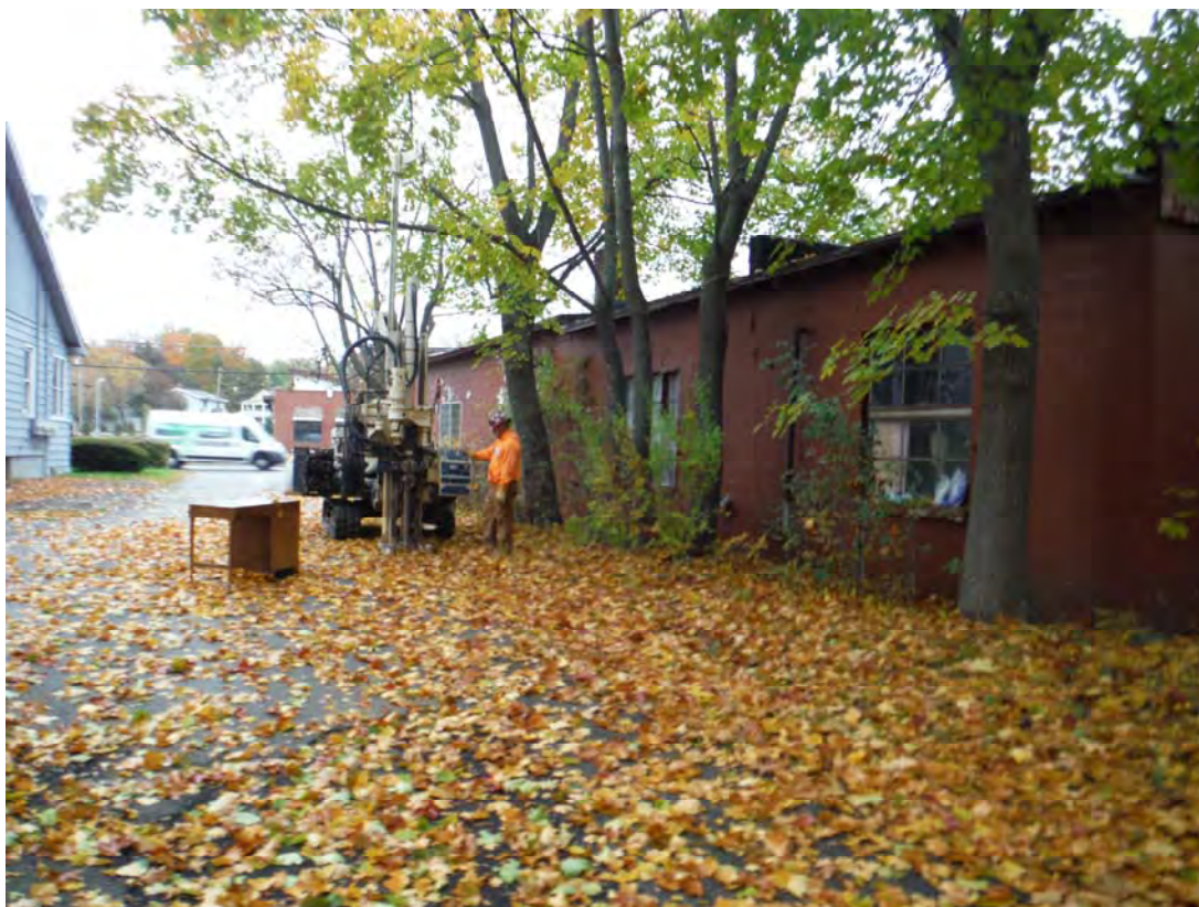
Photograph #2 – Advancement of soil boring SB-2 (monitoring well MW-2) at subject Property on October 20, 2015. Facing northerly.
