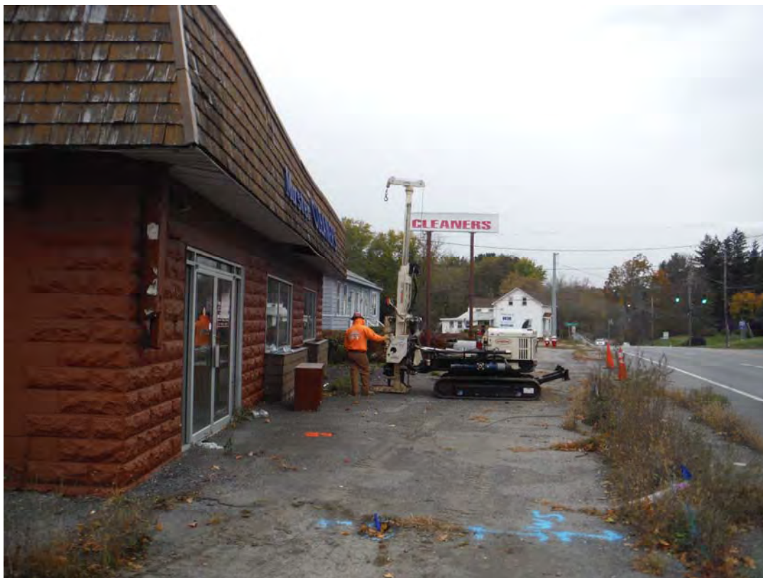
Photograph #1 – Advancement of soil boring SB-1 (monitoring well MW-1) at subject Property on October 20, 2015. Facing westerly.
