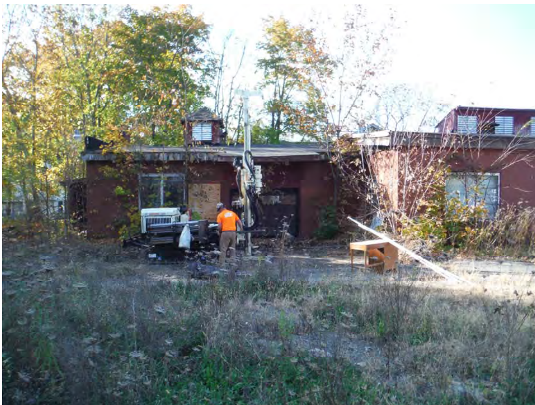
Photograph #4 – Advancement of soil boring SB-4 (monitoring well MW-4) at subject Property on October 20, 2015. Facing westerly.
