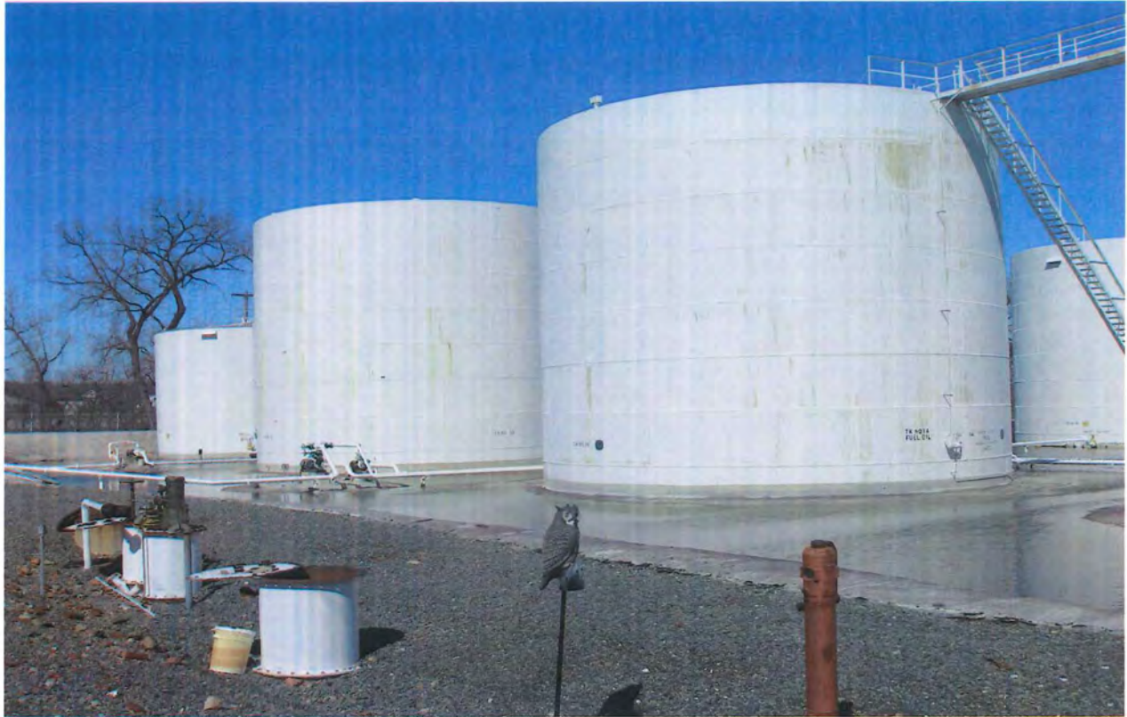
9. View showing the synthetic liner on the ground, in the containment area, around the northern most of the bulk tanks on the property.
