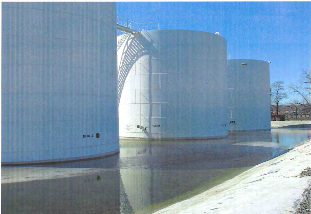
10. View showing the synthetic liner on the ground, in the containment area, around the northern most of the bulk tanks on the property.
