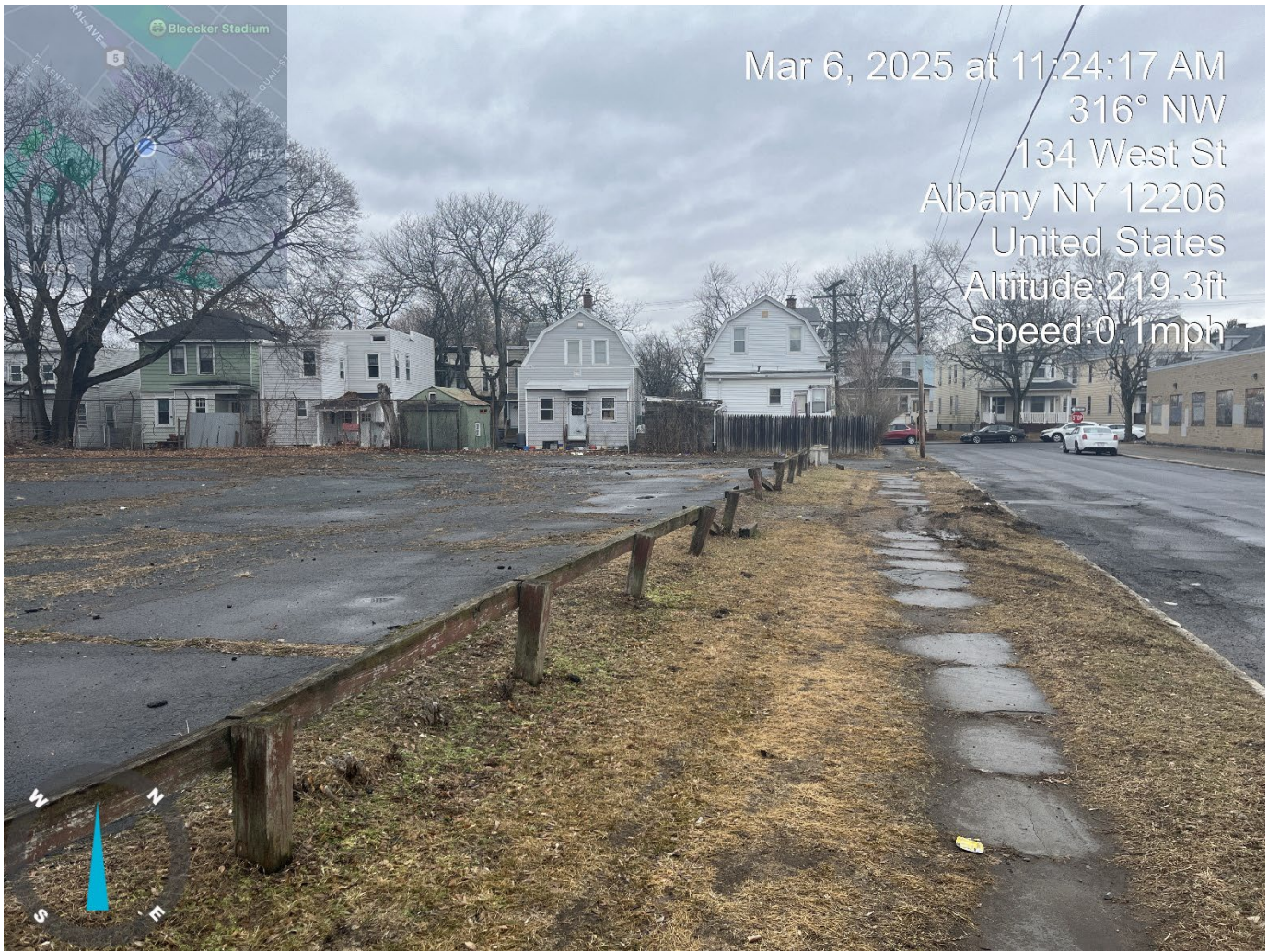
Photo 5 – 134 & 154 West Street facing West
