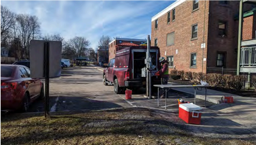
25. View of B-12 location looking northwest.
