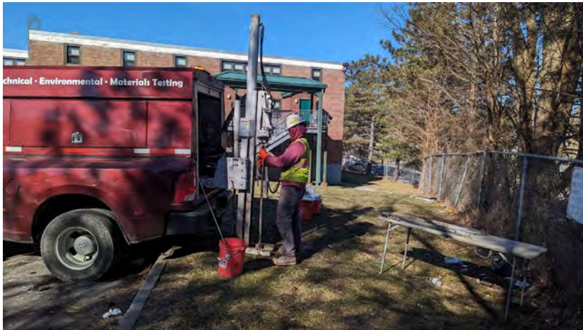
5. View of B-2/MW-2 location, looking northwest
