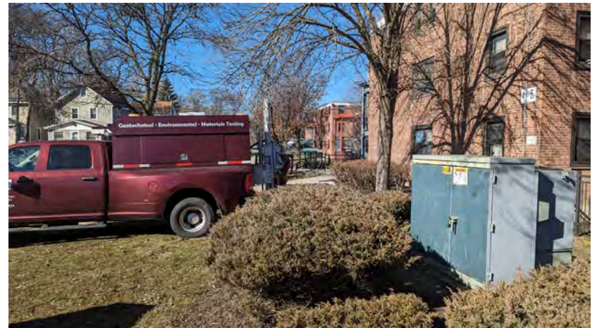
12. View of B-4 location, looking northwest.
