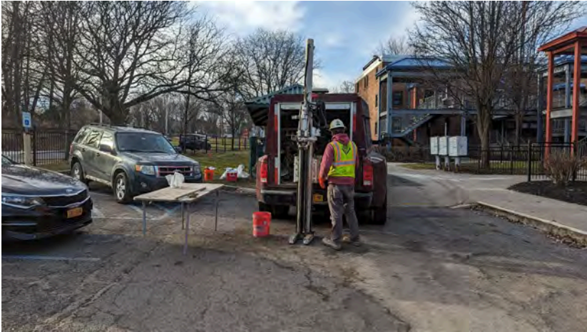
33. View of B-11 location looking northwest.
