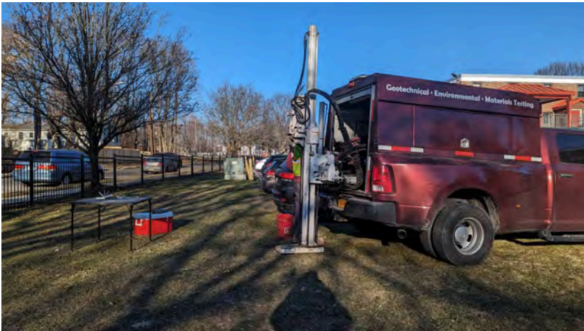
1. View of B-1 location, looking northwest
