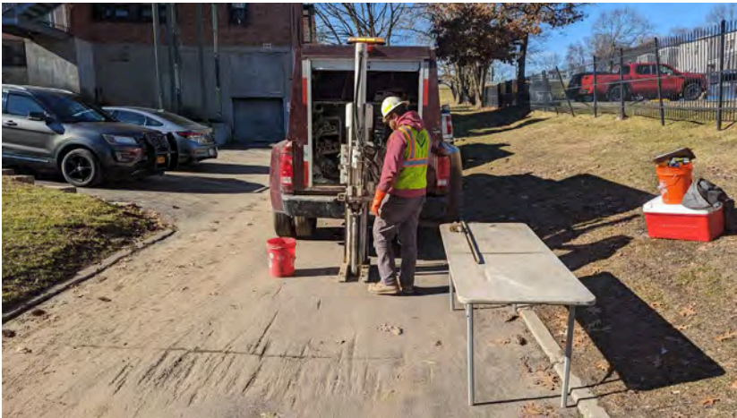
17. View of B-6 location, looking northwest
