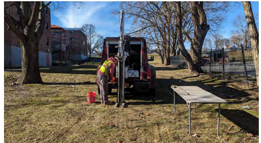
20. View of B-7, looking northwest
