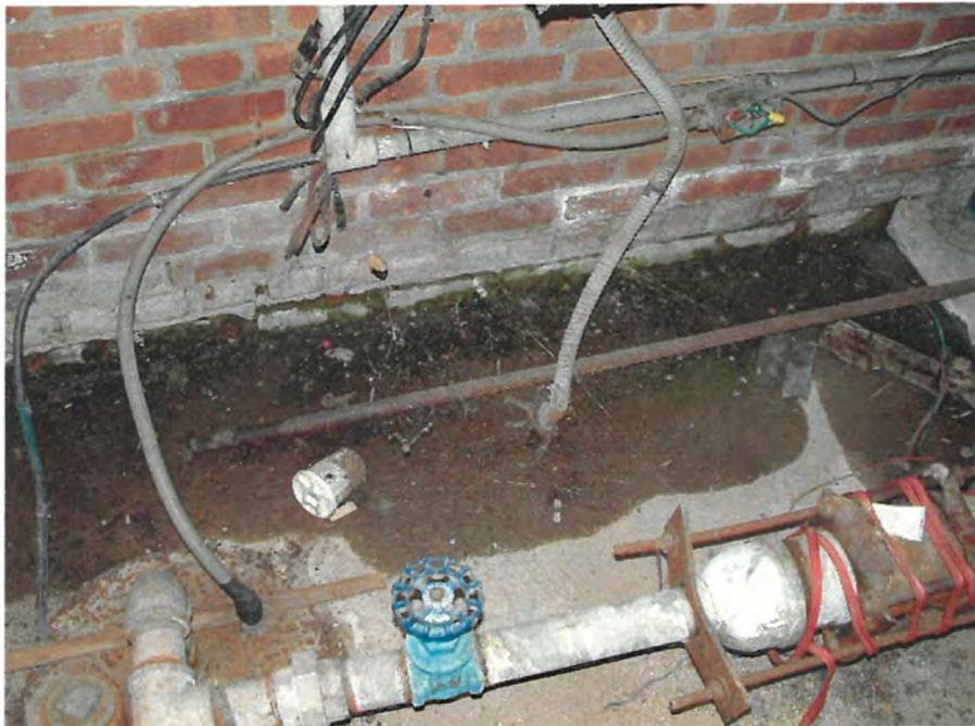
**Photo #8:** Floor of the water pump building, showing hydrocarbon staining on the floor under the previously leaking transformer.
