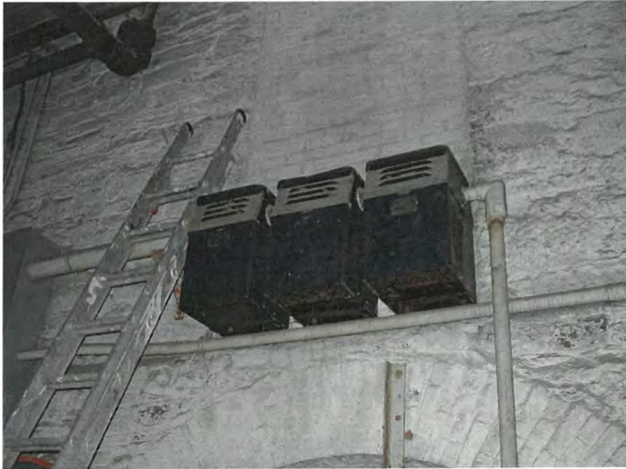
**Photo #9:** The three active transformers in Building 'B', which do not appear to have leaked.
