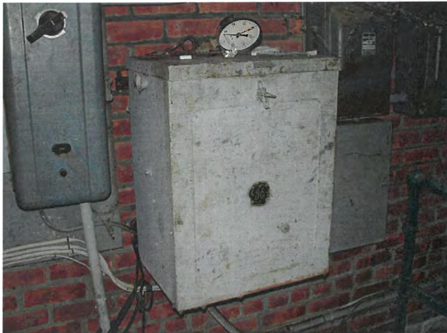
**Photo #7:** Previously leaking inactive transformer located in the vacant water pump building.
