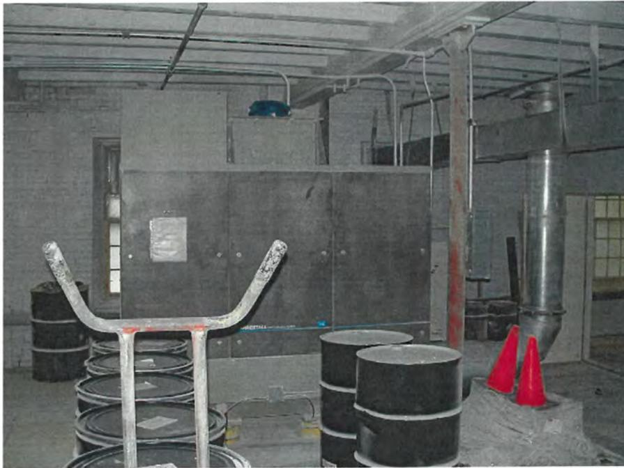
**Photo #3:** One of the three dust collectors on the 2<sup>nd</sup> Floor of Building 'C'.
