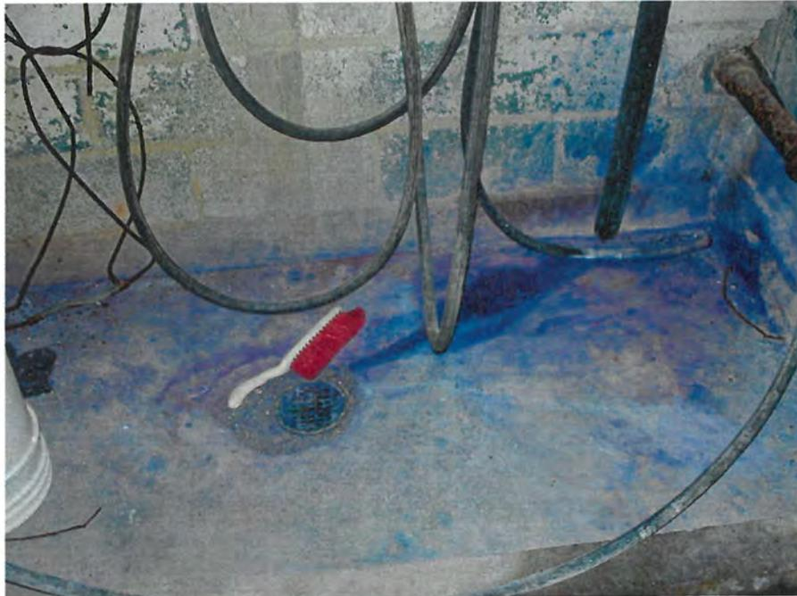
**Photo #1:** A slop sink in the first floor bathroom of Building 'C', showing staining by cleaning agents for Baralyme removal.
