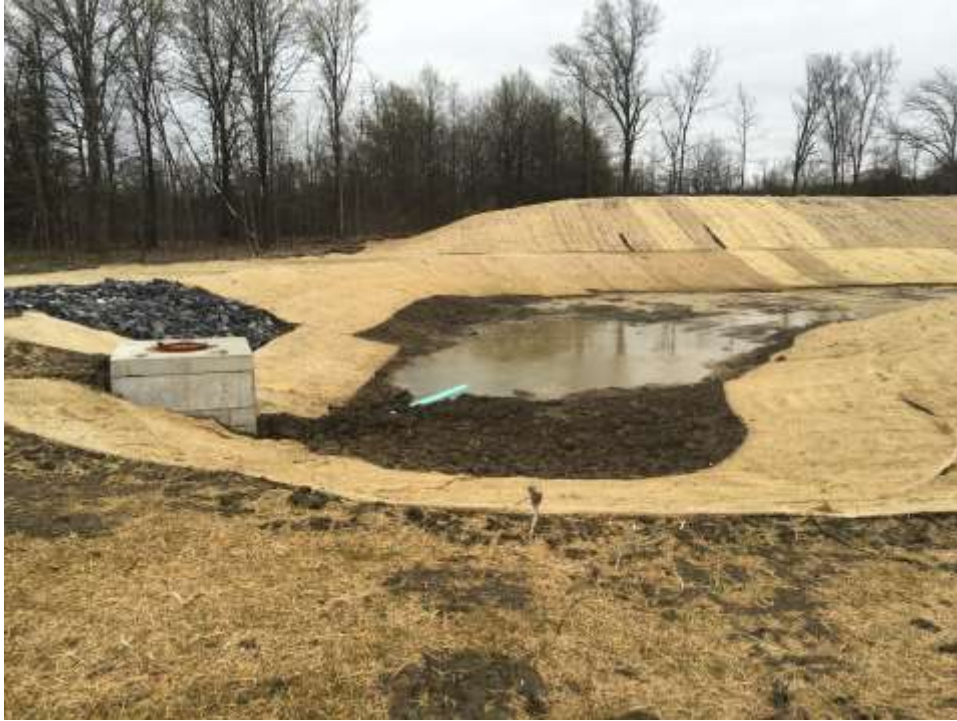
Photograph 21: A new facility stormwater settling basin was constructed adjacent to and north of the Brownfield Cleanup Area Site as a component of the facility redevelopment project. Photograph facing north.
