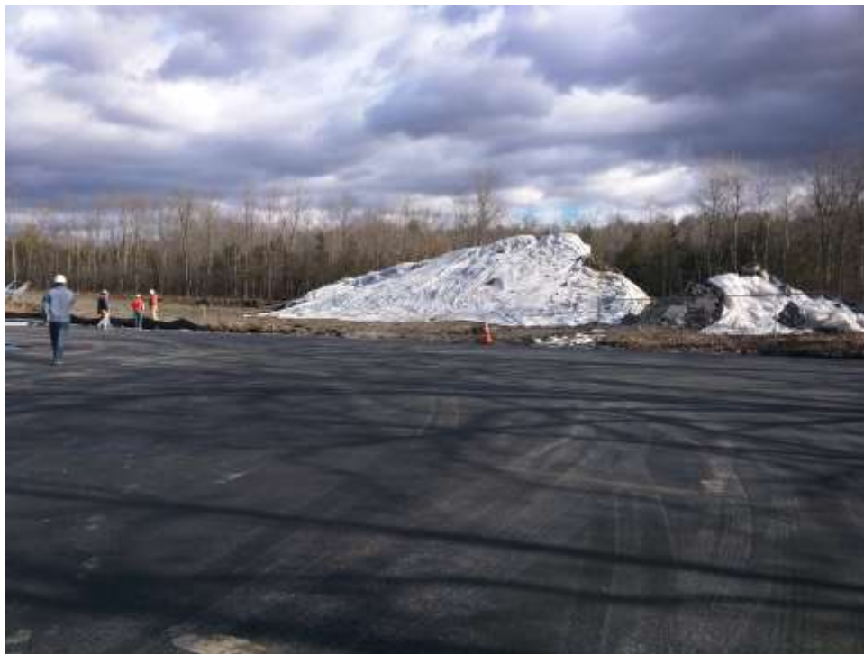
Photograph 14: Excavated impacted soil was consolidated in the vicinity of the concrete debris stockpile area (photograph facing east). Stockpiles were covered with polyethylene sheeting at the end of daily activities.
