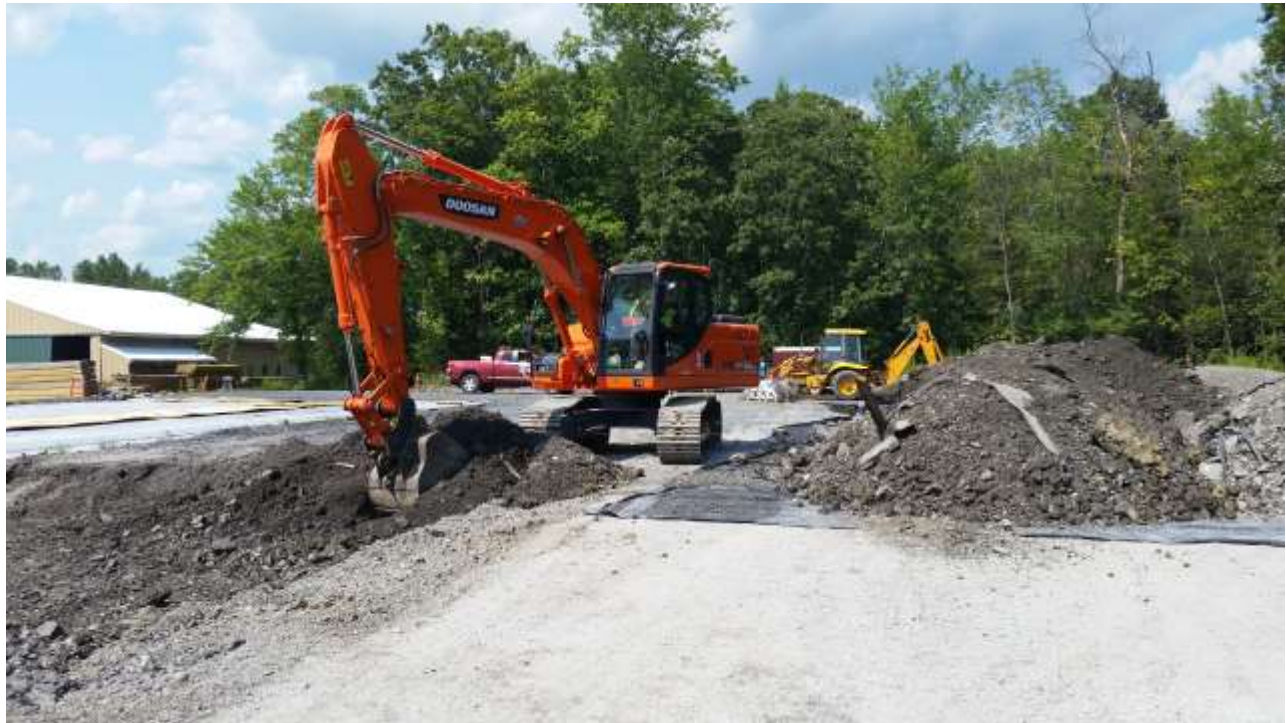
Photograph 2: Excavated impacted soil was stockpiled in designated areas on a layer of polyethylene sheeting.
