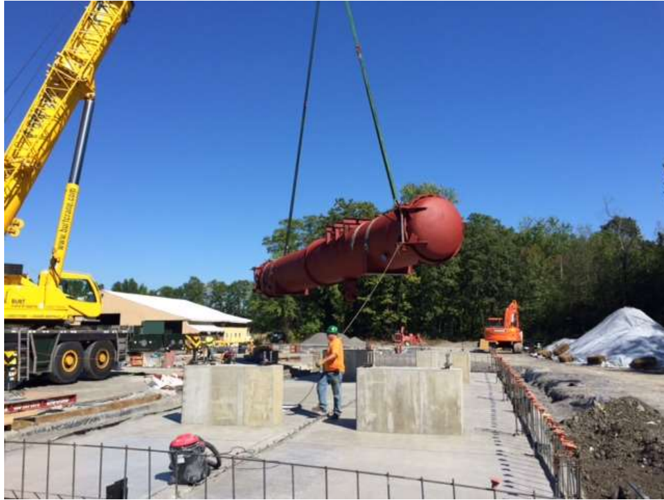
Photograph 9: New industrial wood treatment cylinders were installed.
