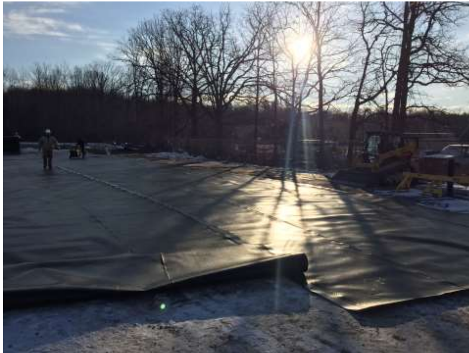
Photograph 12: Construction road fabric was used as a demarcation layer beyond the footprint of the new process building and within the footprint of the Site.
