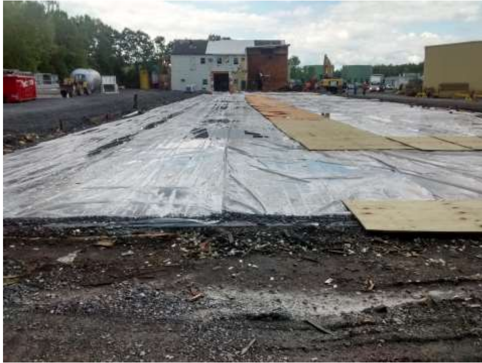
Photograph 1: The concrete drip pad was isolated using polyethylene sheeting and plywood. The drip pad was later sealed with an acrylic-based liquid polymer following excavation activities.
