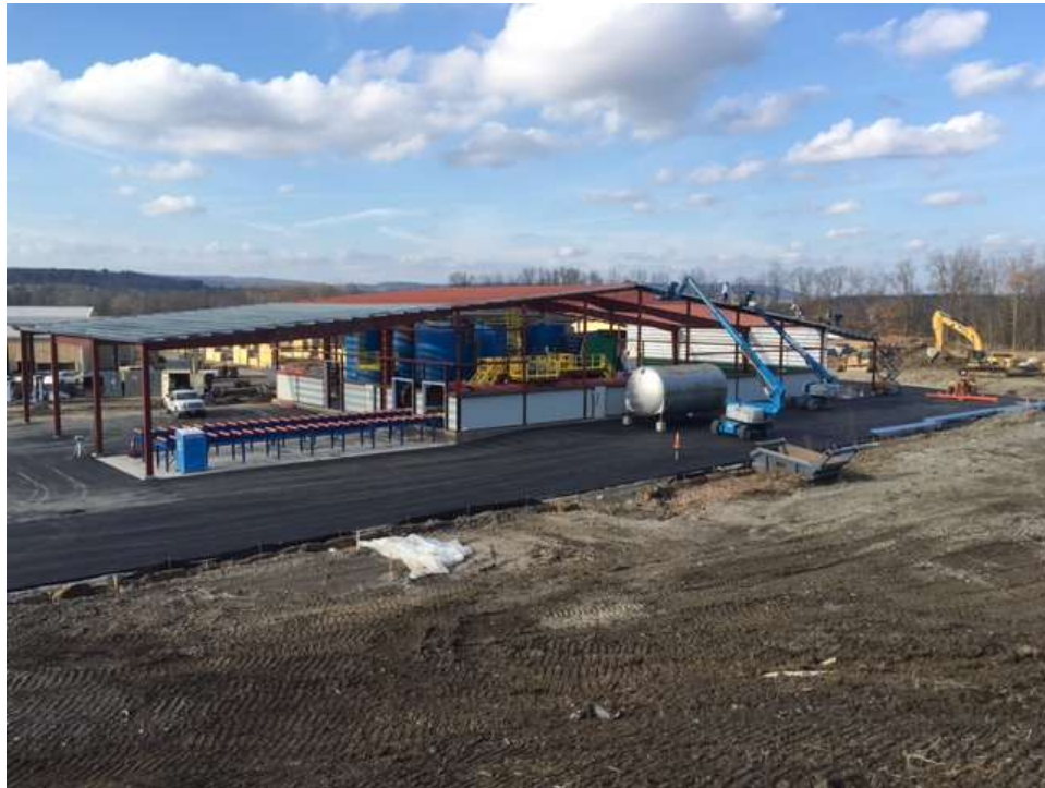
Photograph 16: Construction of the new process building was conducted concurrently with remedial activities. Asphalt paving is an integral part of the protective cover.
