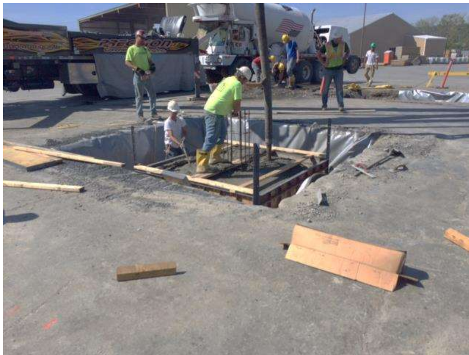
Photograph 8: Polyethylene lined excavations were maintained throughout the building erection sequence.
