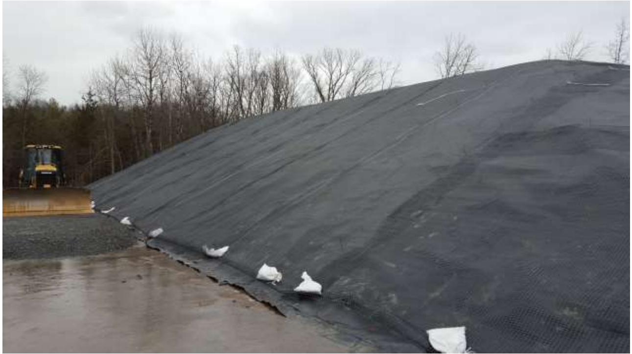
Photograph 17: Impacted soil and concrete comprising the aesthetic berm was encapsulated within an impermeable geomembrane. Recycled concrete aggregate obtained from a NYSDEC registered recycling facility and clean stone was placed over the storage yard expansion area.
