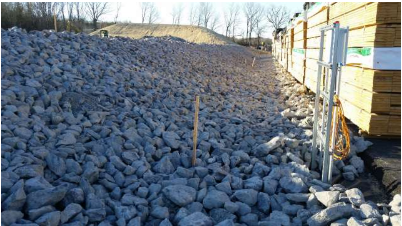
Photograph 20: A minimum of one (1) foot of clean imported riprap was placed between the original Northeast Treaters facility and the newly constructed expansion area. Photograph facing south.
