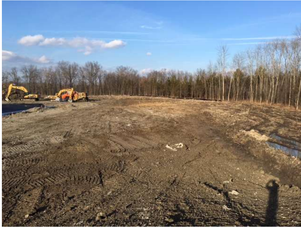
Photograph 13: The undeveloped woodland area east of the new process building was cleared and grubbed to expand product storage capacity (photograph facing north).
