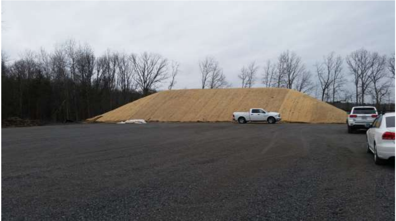
Photograph 19: Erosion control matting was placed over the one (1) foot soil cover of the noise abatement berm.
