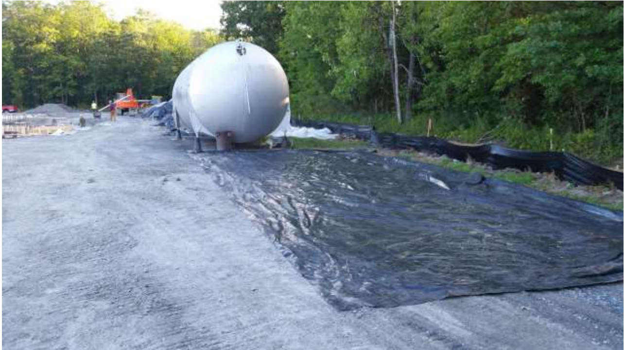
Photograph 3: Designated impacted soil stockpile areas were located along eastern portion of the developed Site. Erosion and sediment control measures were established along the perimeter of the construction area.
