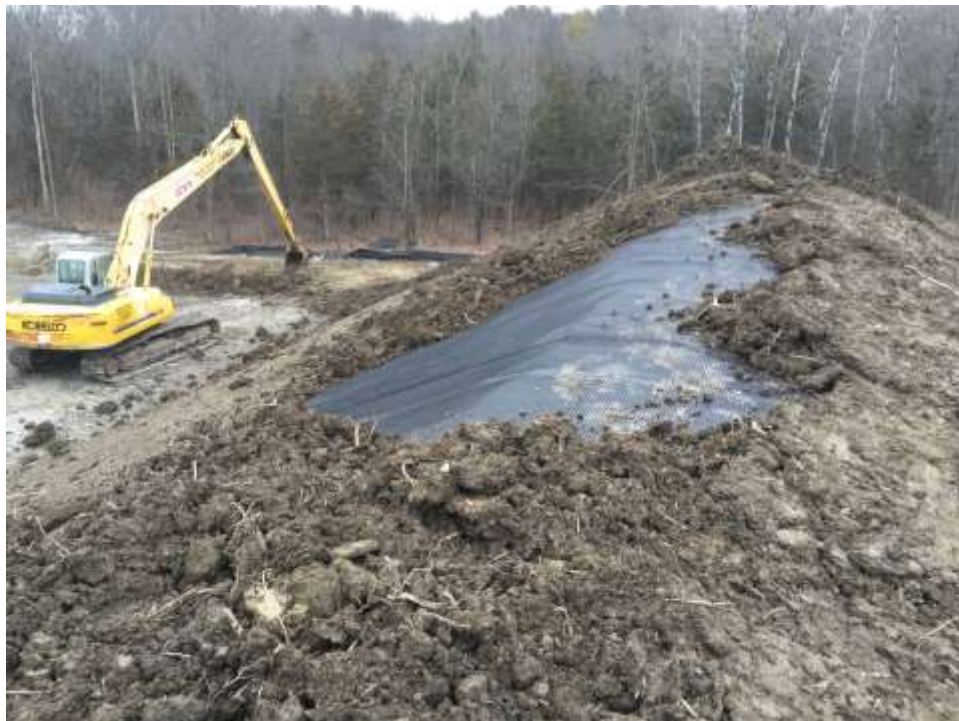
Photograph 18: A minimum of one (1) foot of clean imported soil was placed over the aesthetic berm and above the impermeable geomembrane.
