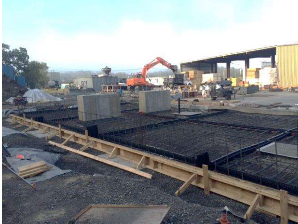
Photograph 7: Formwork for structural components was assembled within excavation areas.
