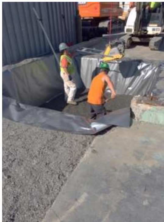
Photograph 6: Worker exposure to impacted soil within excavation areas was limited by polyethylene sheeting and clean stone.
