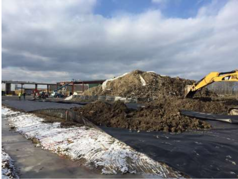
Photograph 15: Consolidated impacted soil and stockpiled concrete debris were used to construct an aesthetic berm on the southernmost portion of the storage yard expansion area.
