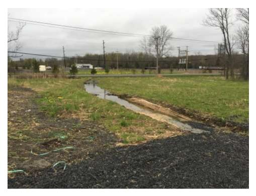
Photograph 22: The offsite drainage exit swale located south of the existing facility stormwater settling basin was modified during remedial activities.
