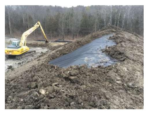
Photograph 18: A minimum of one (1) foot of clean imported soil was placed over the aesthetic berm and above the impermeable geomembrane.
