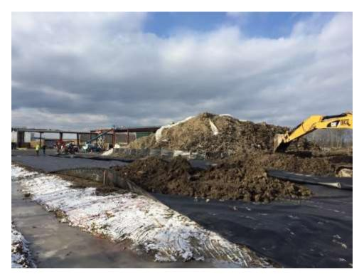
Photograph 15: Consolidated impacted soil and stockpiled concrete debris were used to construct an aesthetic berm on the southernmost portion of the storage yard expansion area.
