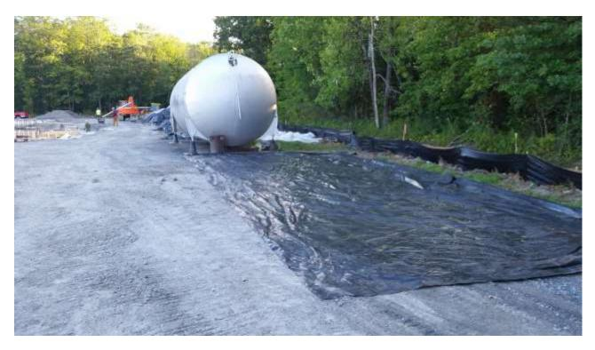
Photograph 3: Designated impacted soil stockpile areas were located along eastern portion of the developed Site. Erosion and sediment control measures were established along the perimeter of the construction area.
