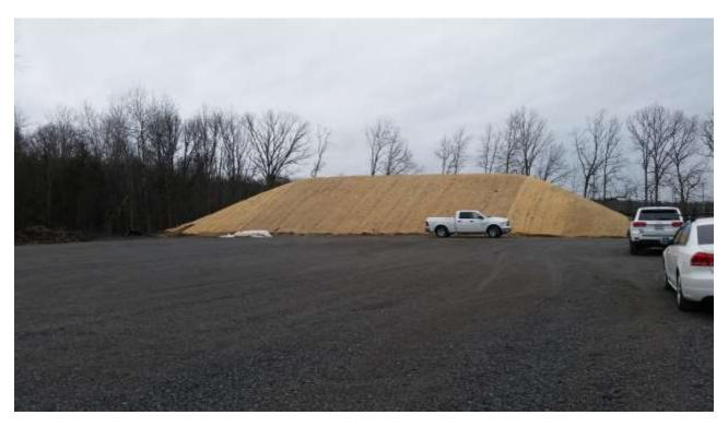
Photograph 19: Erosion control matting was placed over the one (1) foot soil cover of the noise abatement berm.
