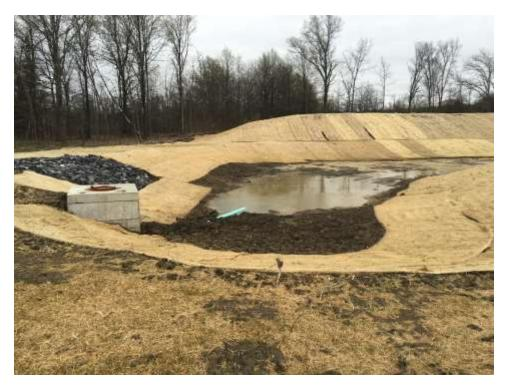
Photograph 21: A new facility stormwater settling basin was constructed adjacent to and north of the Brownfield Cleanup Area Site as a component of the facility redevelopment project. Photograph facing north.
