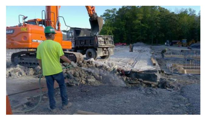
Photograph 4: Potable water was used for dust control, as needed.
