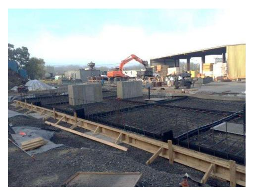
Photograph 7: Formwork for structural components was assembled within excavation areas.
