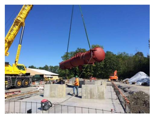
Photograph 9: New industrial wood treatment cylinders were installed.
