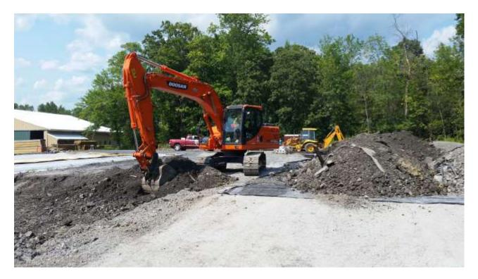
Photograph 2: Excavated impacted soil was stockpiled in designated areas on a layer of polyethylene sheeting.
