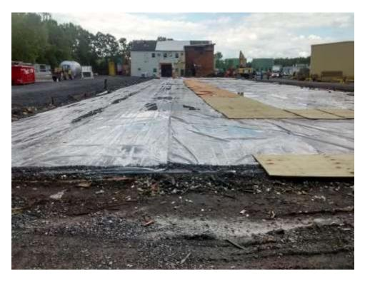
Photograph 1: The concrete drip pad was isolated using polyethylene sheeting and plywood. The drip pad was later sealed with an acrylic-based liquid polymer following excavation activities.
