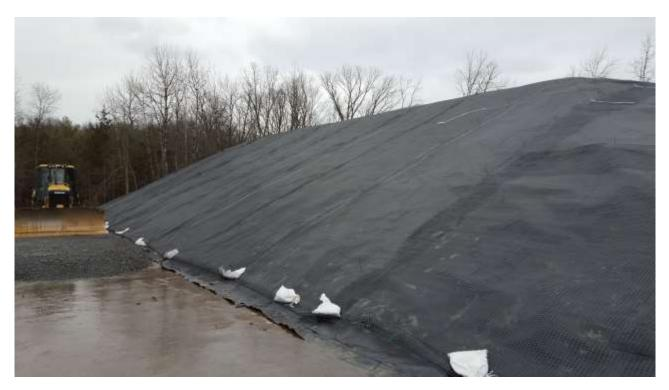
Photograph 17: Impacted soil and concrete comprising the aesthetic berm was encapsulated within an impermeable geomembrane. Recycled concrete aggregate obtained from a NYSDEC registered recycling facility and clean stone was placed over the storage yard expansion area.
