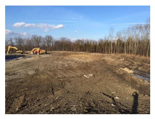
Photograph 13: The undeveloped woodland area east of the new process building was cleared and grubbed to expand product storage capacity (photograph facing north).
