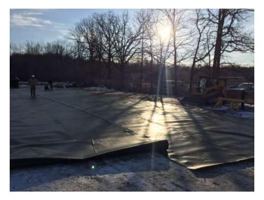
Photograph 12: Construction road fabric was used as a demarcation layer beyond the footprint of the new process building and within the footprint of the Site.
