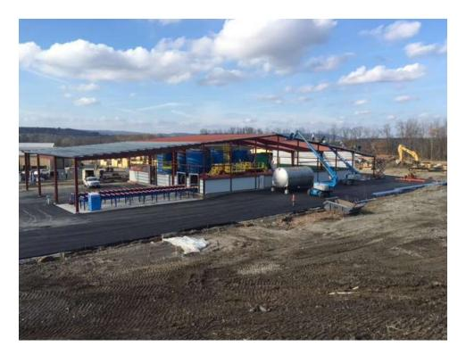
Photograph 16: Construction of the new process building was conducted concurrently with remedial activities. Asphalt paving is an integral part of the protective cover.
