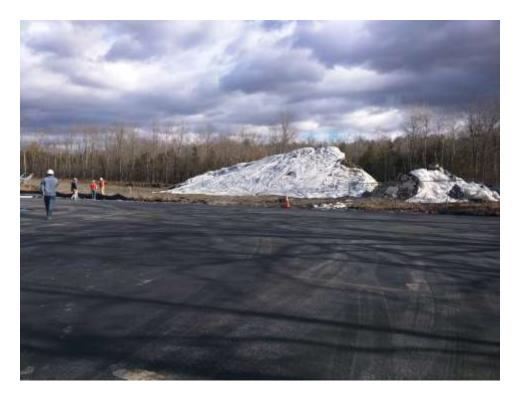
Photograph 14: Excavated impacted soil was consolidated in the vicinity of the concrete debris stockpile area (photograph facing east). Stockpiles were covered with polyethylene sheeting at the end of daily activities.
