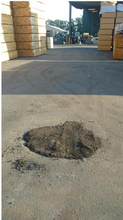
Photograph 10: Asphalt depression shown in Photographs 1 and 2 was repaired on August 29, 2018.
