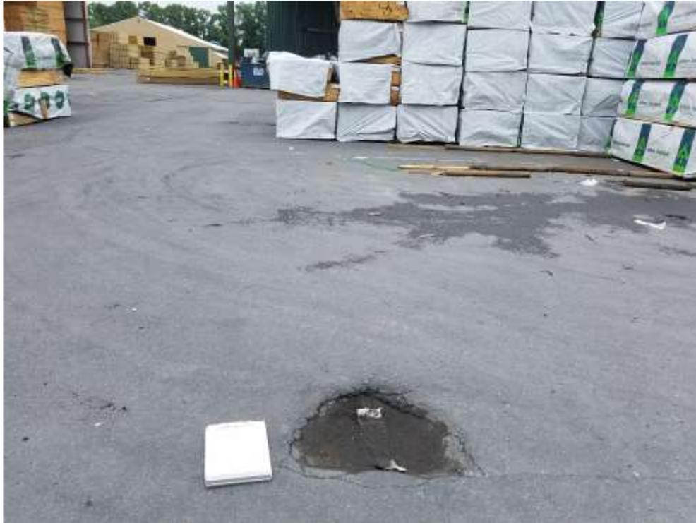
Photograph 1: Depression in asphalt pavement at southwestern portion of Site.
