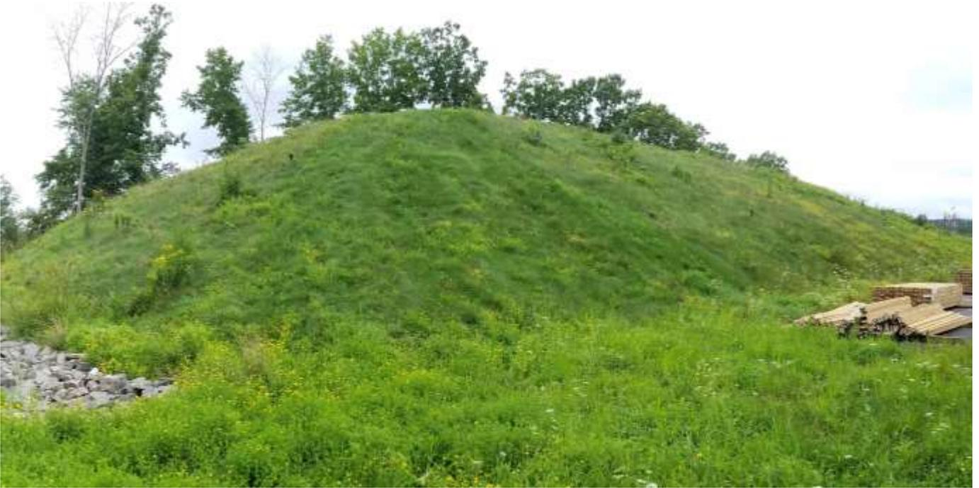
Photograph 5: Abatement berm, facing southwest. Soil cover in acceptable condition.
