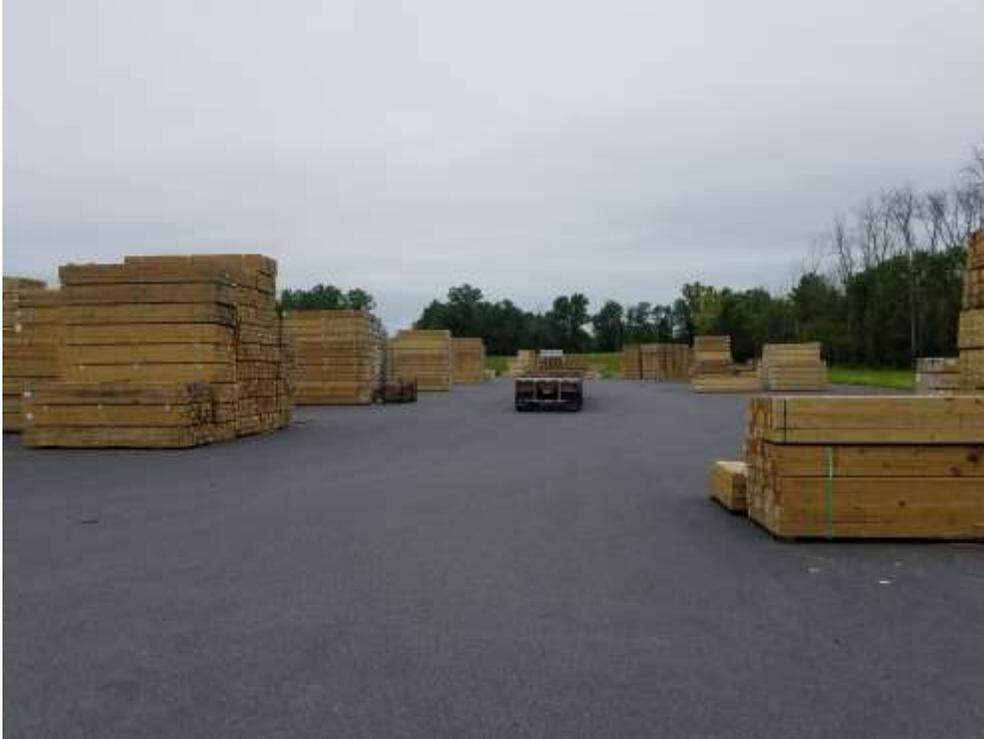
Photograph 3: Asphalt pavement at eastern lumber storage area in acceptable condition.
