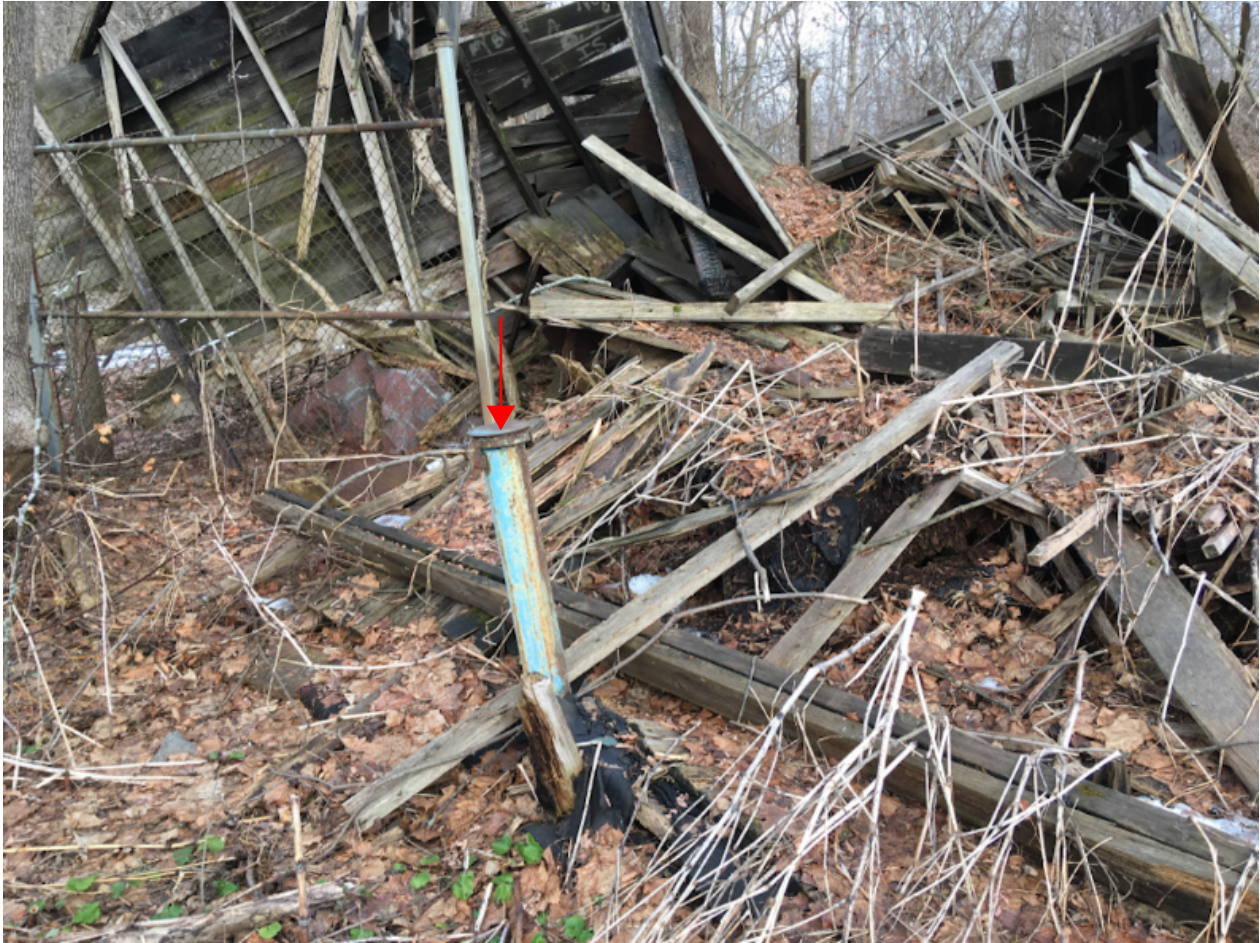
10. MW-2 - Facing North
