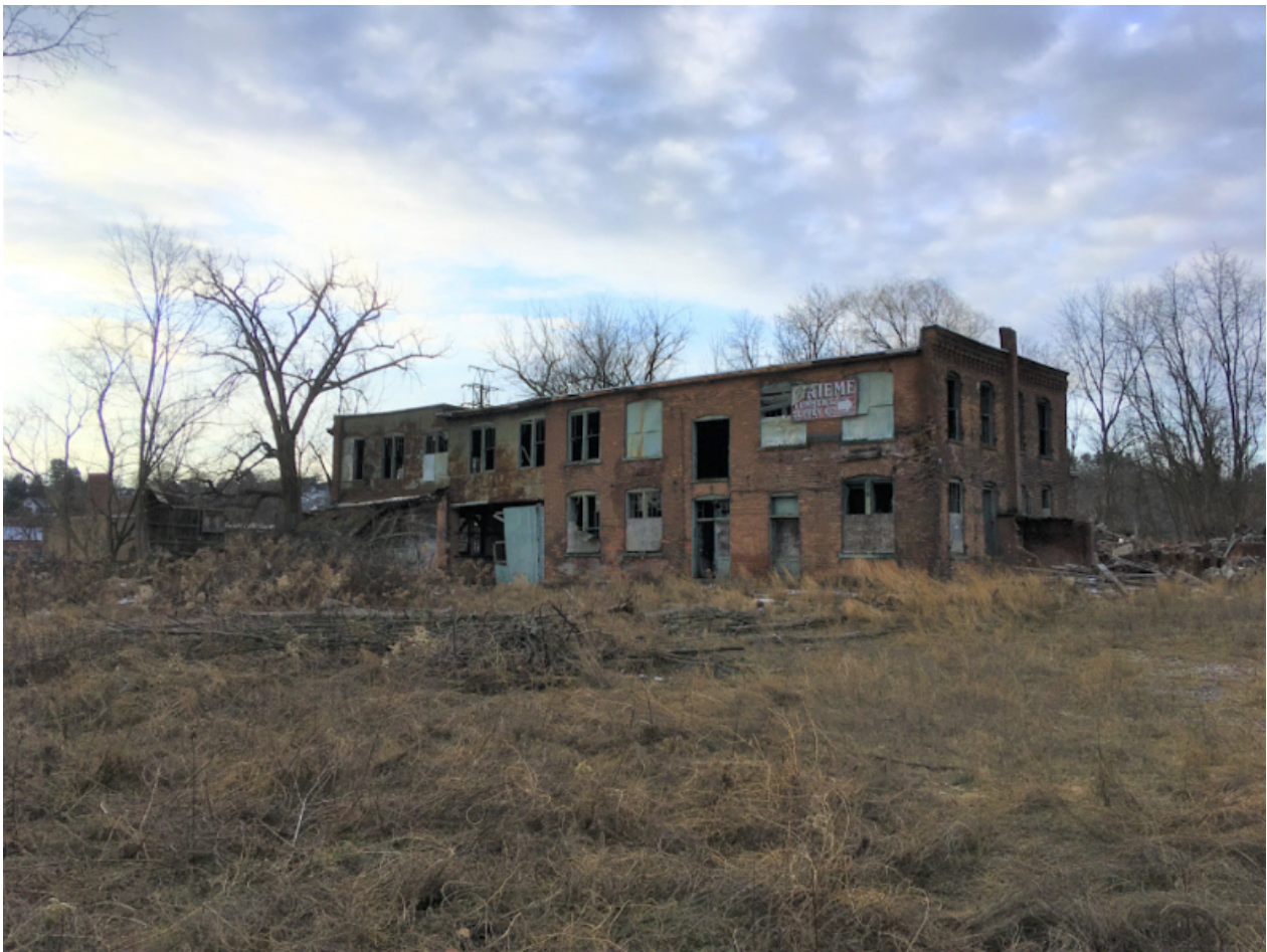
1. Building A Overview - Facing Southwest
