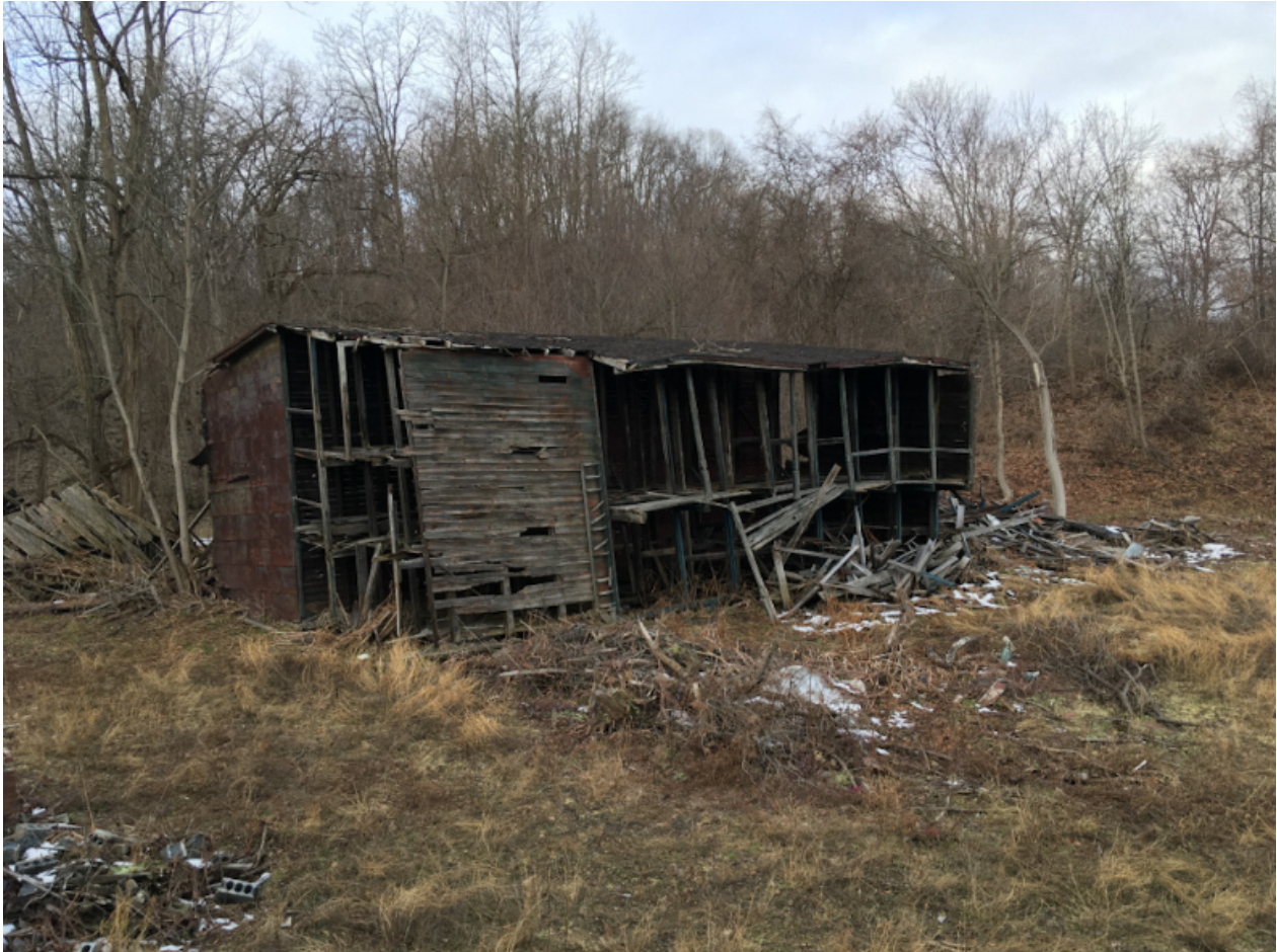
2. Building B Overview - Facing West
