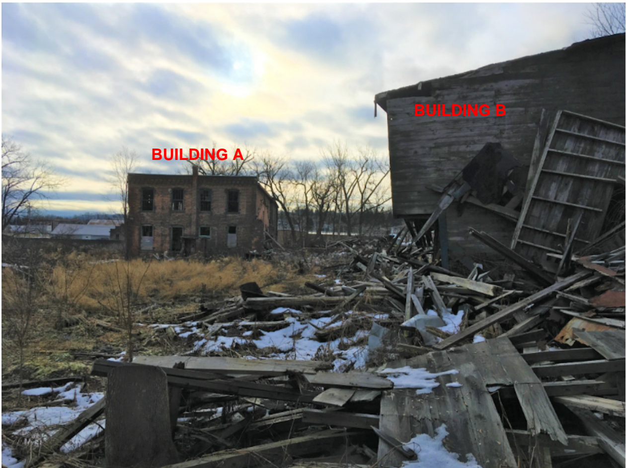
14. Building B and A - Facing South
