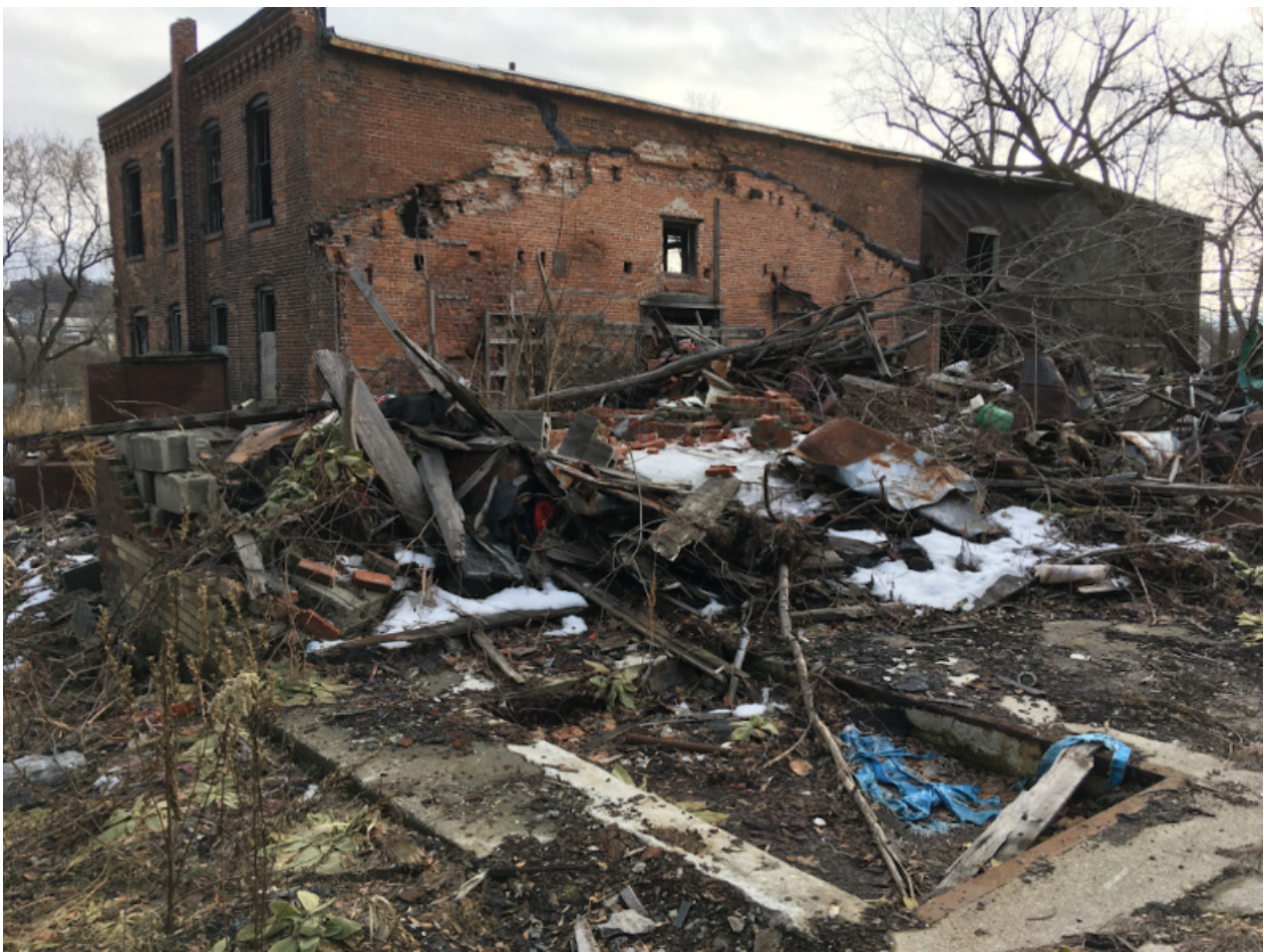
3. Building A Demo Area - Facing Southeast
