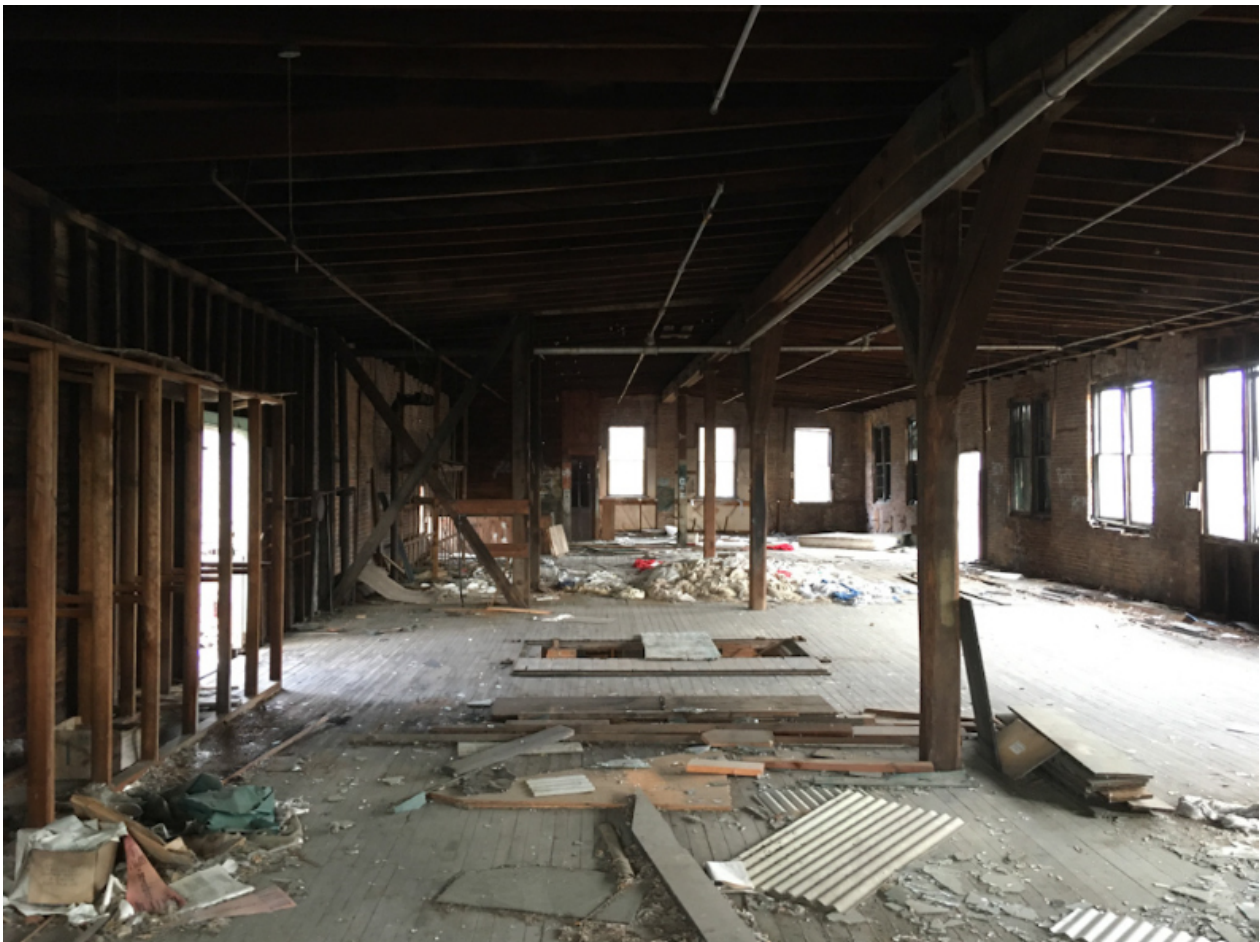
6. Second Story Interior, Building A - Facing North
