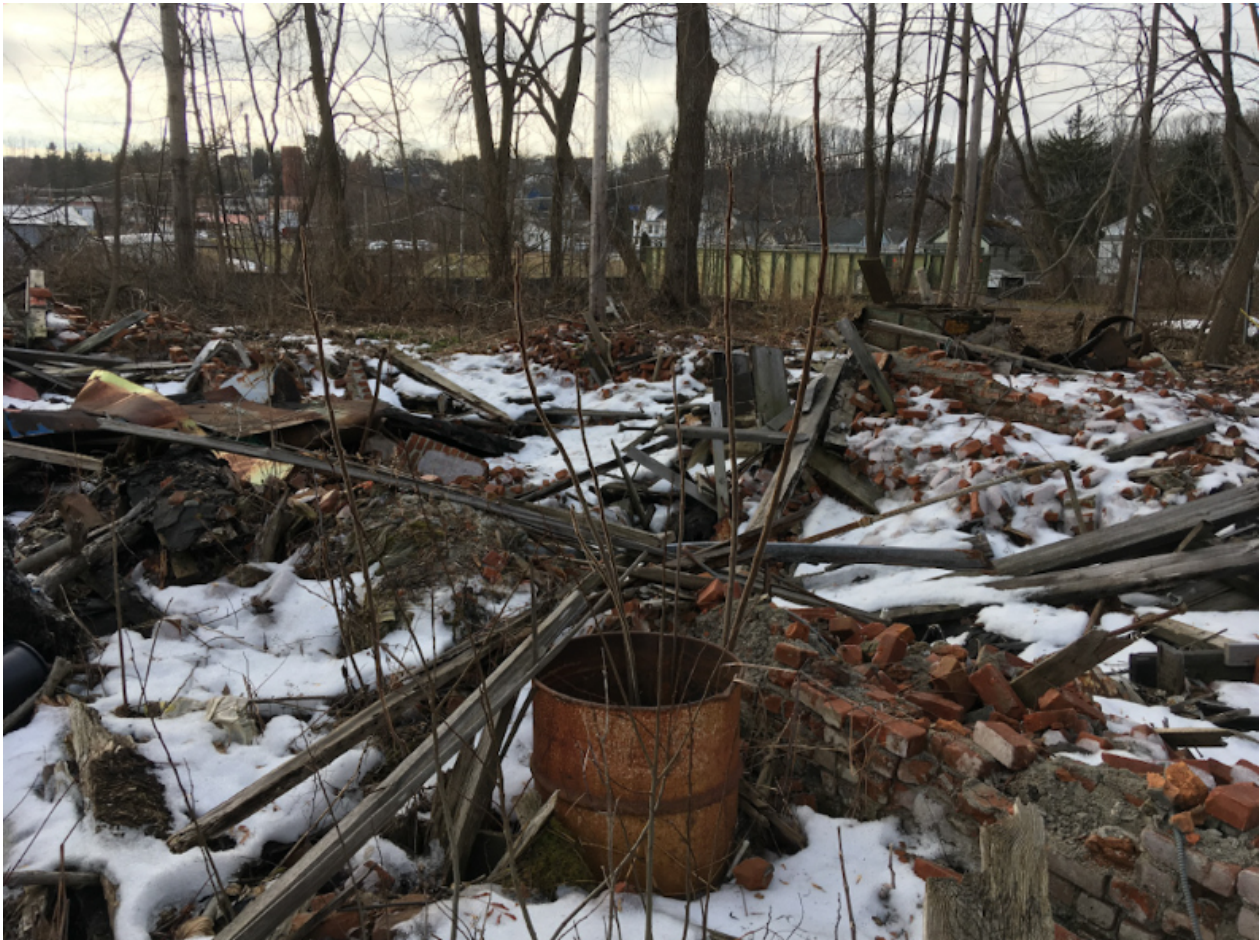
4. Building A Demo Area - Facing West
