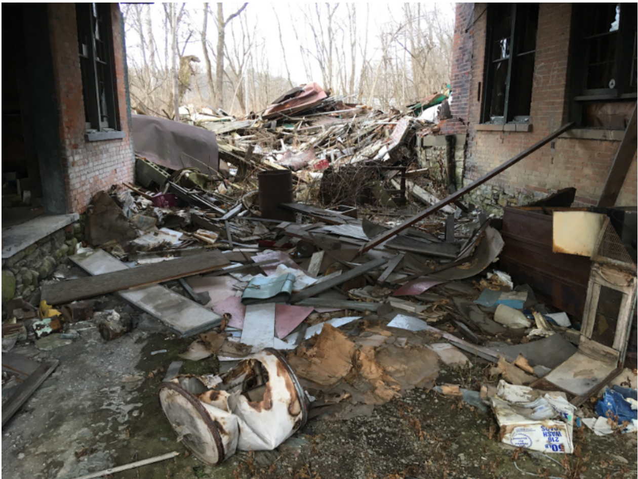
5. Debris and Demo Area Around Building A - Facing West
