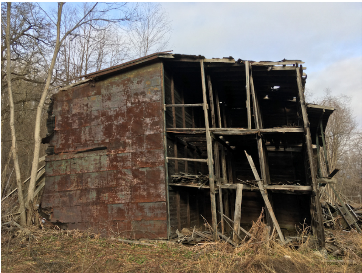
7. Building B Exterior - Facing North
